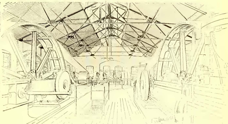
The above illustration is taken direct from a photograph, and shows the interior of a dynamo room, the roof of which was designed and built by us for the Worcester, Leicester & Spencer Street Railway Co., at Worcester, Mass.
