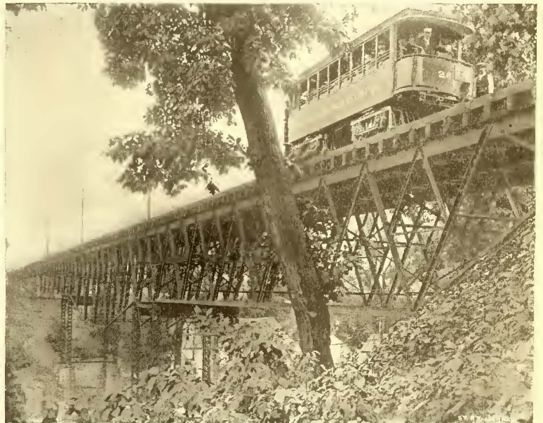
FIG. 6.—STONY RUN VIADUCT—LAKE ROLAND ELEVATED RAILWAY.
