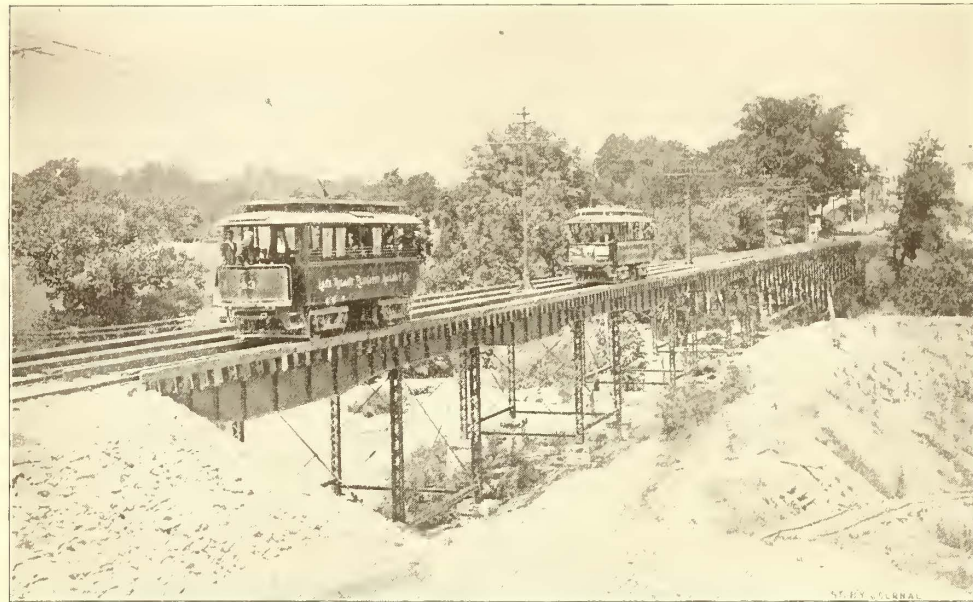
FIG. 7.—STONY RUN VIADUCT—LAKE ROLAND ELEVATED RAILWAY
