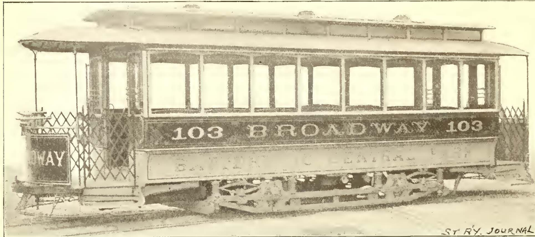
FIG 4.—CABLE CAR—BROADWAY CABLE RAILWAY, NEW YORK.
