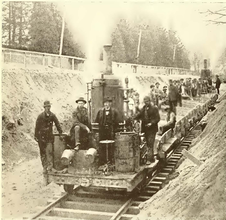
FIG. 3.—CHANGING GRADE, YORK ROAD—CITY & SUBURBAN RAILWAY.
