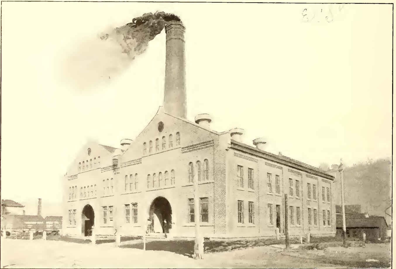
FIG. 1.—POWER STATION—WHEELING ELECTRIC RAILWAY.
