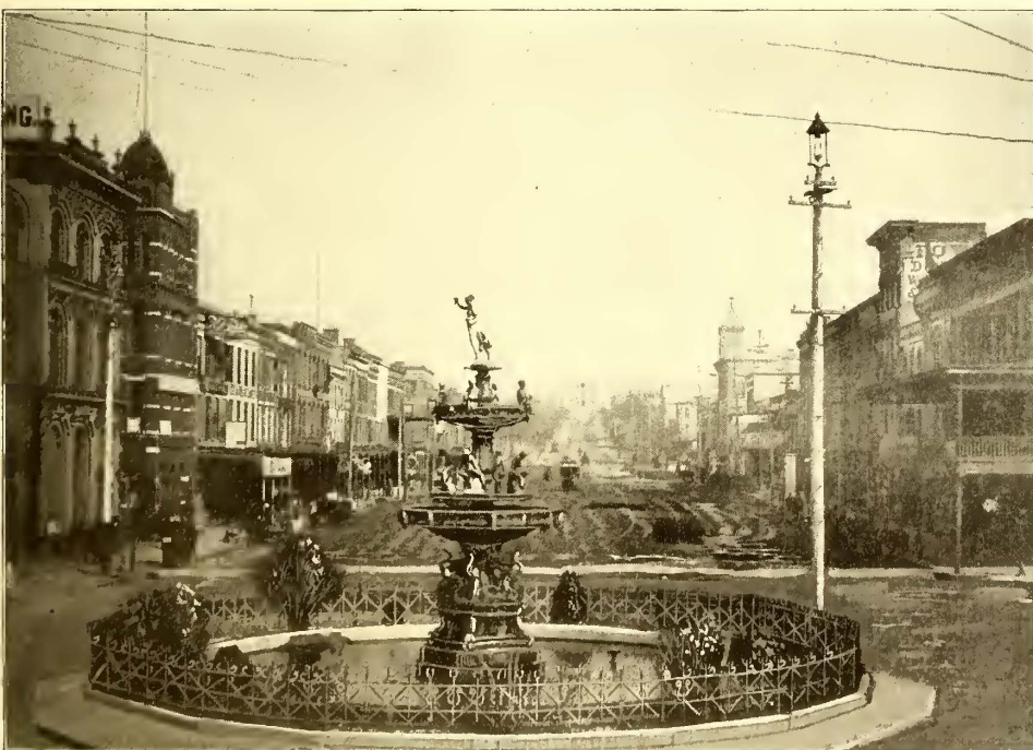
FIG. 1.—VIEW ON DEXTER AVENUE—MONTGOMERY, ALA.
