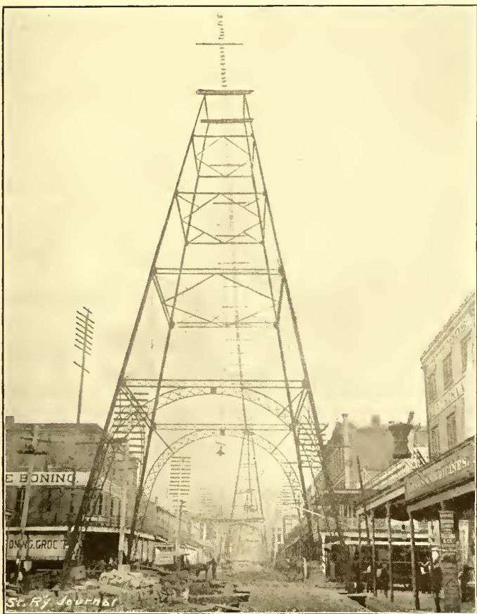
FIG. 13.—TOWERS ERECTED FOR ELECTRIC LIGHTING—NEW ORLEANS.
