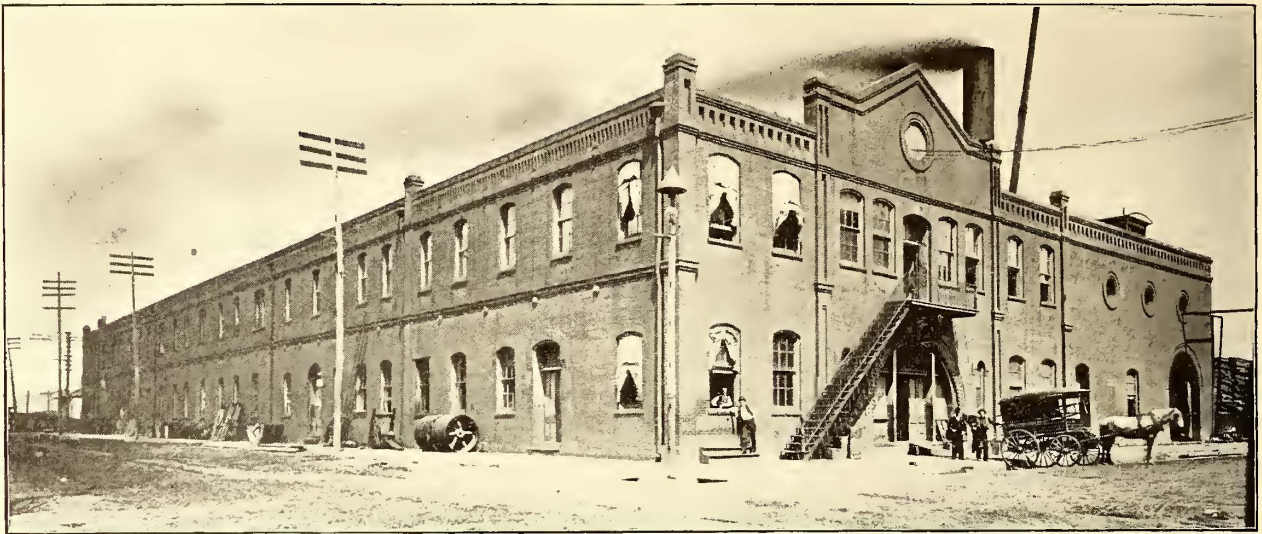
FIG. 7.—EXTERIOR OF STATION—LOUISIANA ELECTRIC LIGHT CO.
