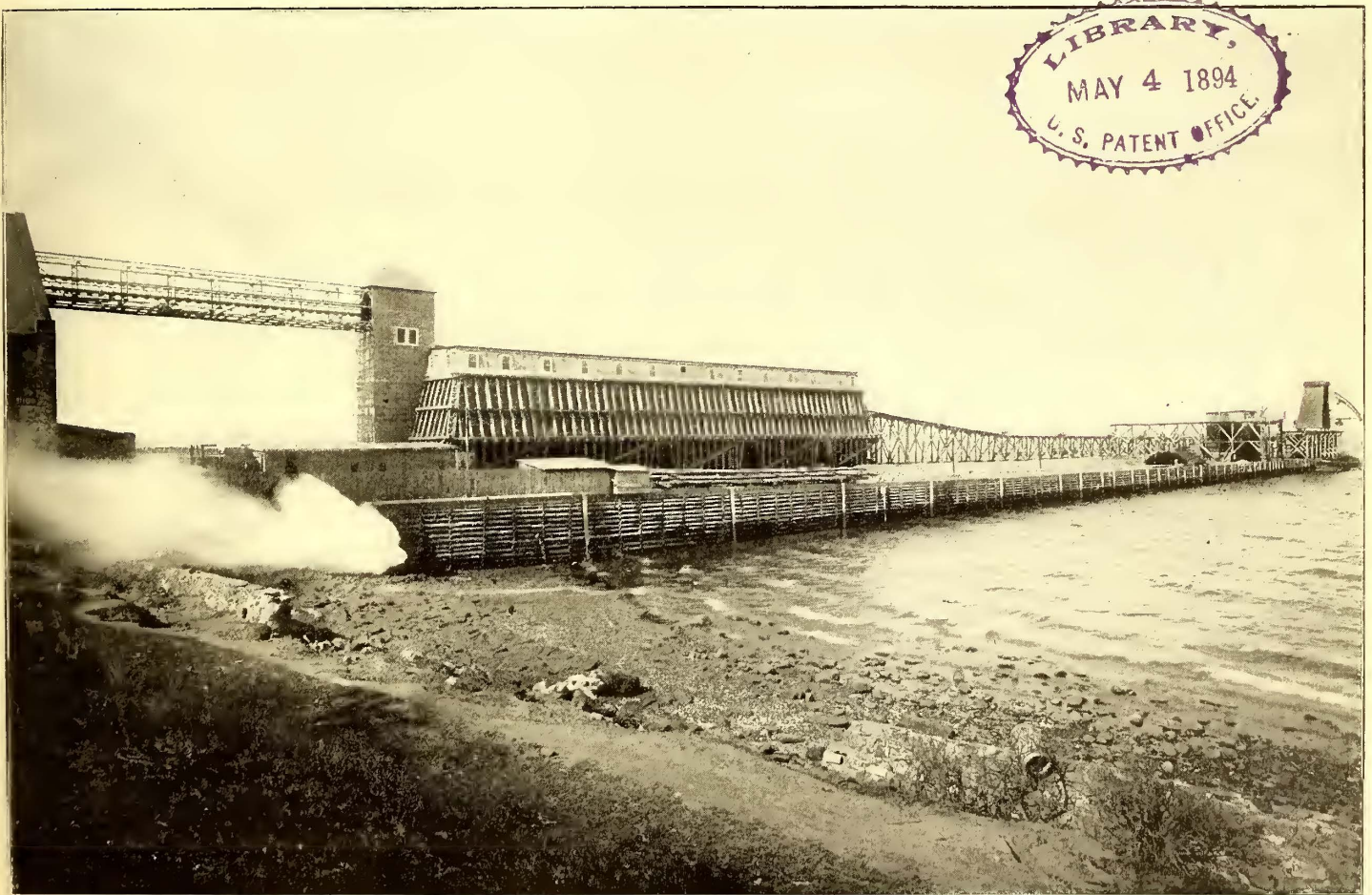
FIG. 1—GENERAL VIEW OF COAL HANDLING APPARATUS—SOUTHERN STATION OF BROOKLYN CITY RAILWAY.
