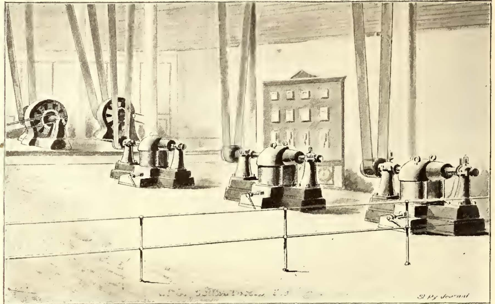
FIG. 8.—SYNCHRONOUS MOTORS OPERATING RAILWAY GENERATORS—PONEMAH MILLS.
