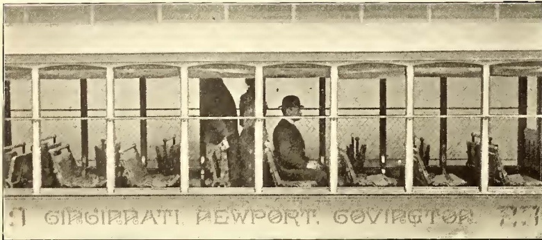
FIGS. 5 AND 6.—OPEN CAR AND FOLDABLE SEATS—CINCINNATI, NEWPORT & COVINGTON RAILWAY.
