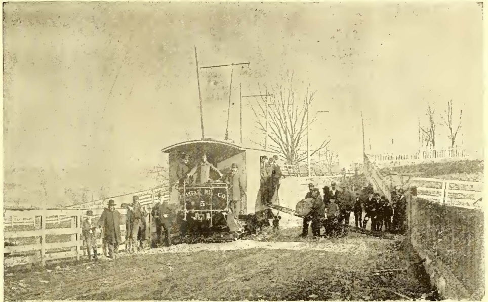
FIG. 2.—ELECTRIC LOCOMOTIVE—CAPITAL RAILWAY, FRANKFORT.
