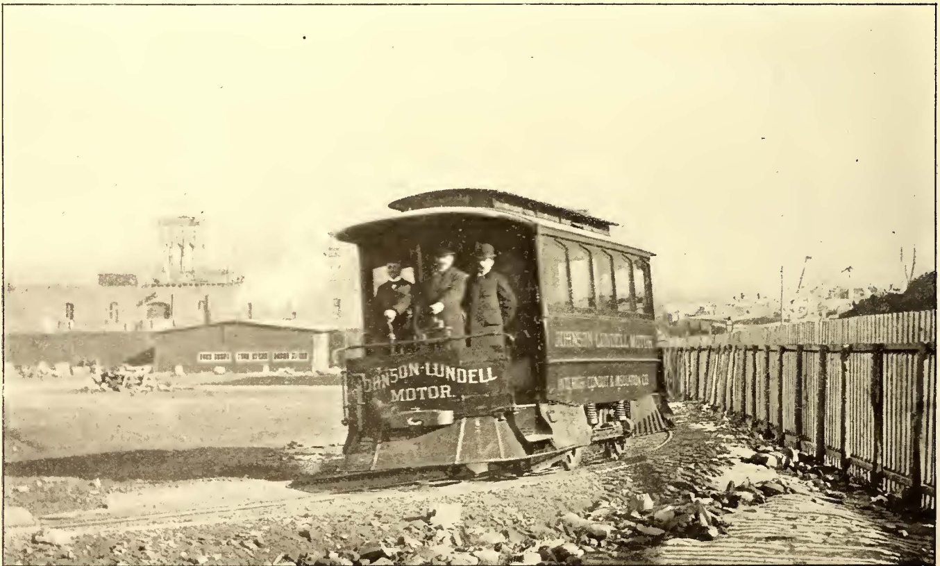
FIG. 2.—CAR MOUNTING GRADE—SURFACE CONTACT RAILWAY SYSTEM.
