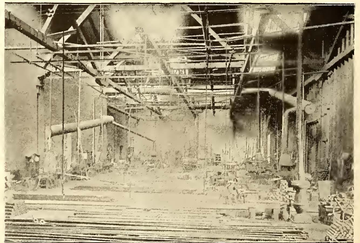
FIG. 3.—SMITH SHOP—WROUGHT IRON BRIDGE CO.
