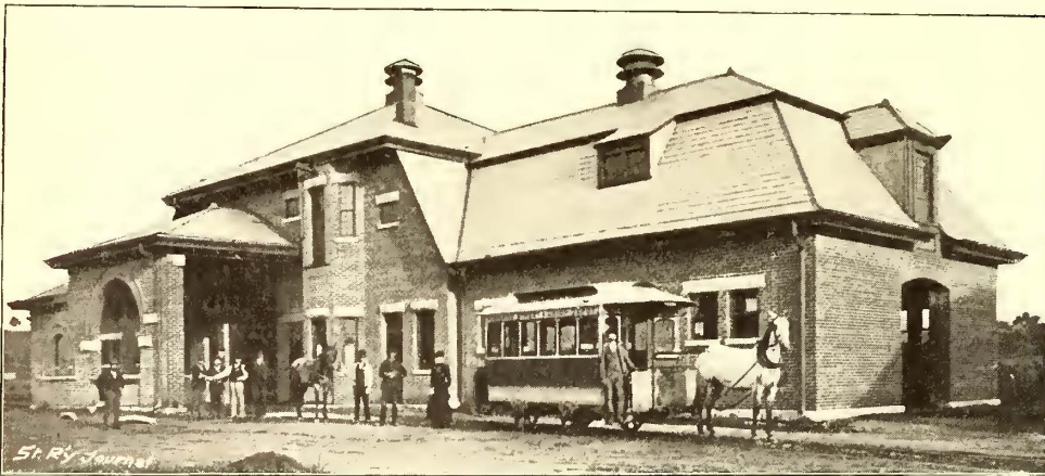
FIG. 4.—ONE OF THE CAR HOUSES—CITY RAILWAY CO., DAYTON.
