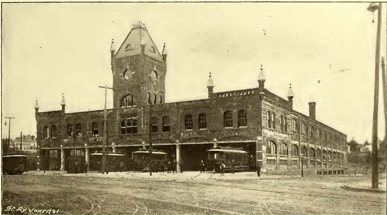
FIG. 1—EXTERIOR OF CAR HOUSE—UNION RAILWAY COMPANY, NEW YORK CITY.
