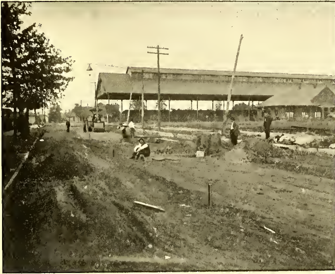
FIRST PROCESS—ROLLING THE ROADBED AFTER EXCAVATION.
