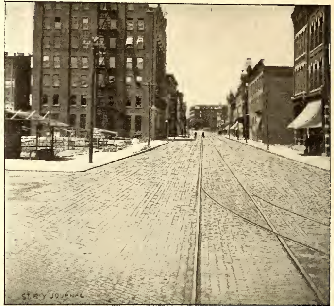
FIG. 2.—T RAIL IN BRICK PAVING—ROANOKE.
