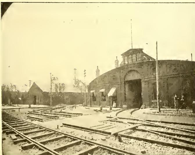
DOUBLE AND SINGLE CURVES AT POWER HOUSE.
