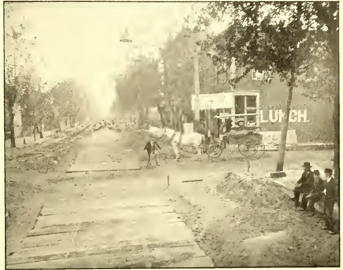
SECOND PROCESS—PREPARING TO RECEIVE THE BROKEN STONE—SETTING STAKES.
