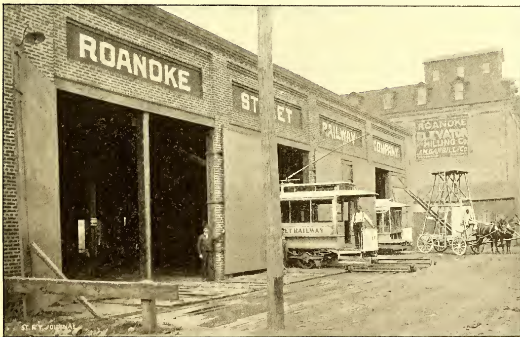
FIG. 4.—CAR HOUSE—ROANOKE STREET RAILWAY CO.
