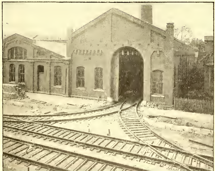
Y CURVES AT POWER HOUSE.
