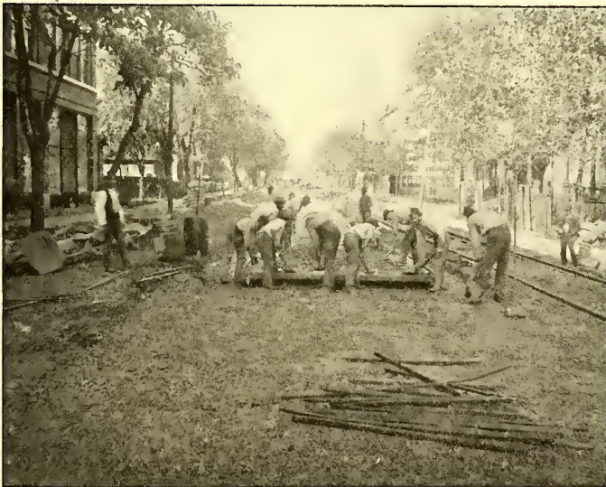
THIRD PROCESS—LAYING THE FIRST EIGHT INCHES OF BROKEN STONE.
