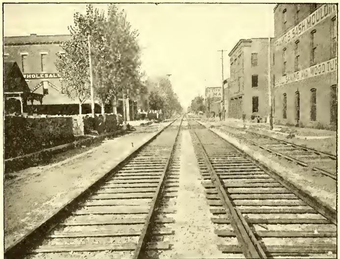
FOURTH PROCESS—TRACK READY FOR TAMPING WITH LAST FOUR INCHES OF BROKEN STONE.
