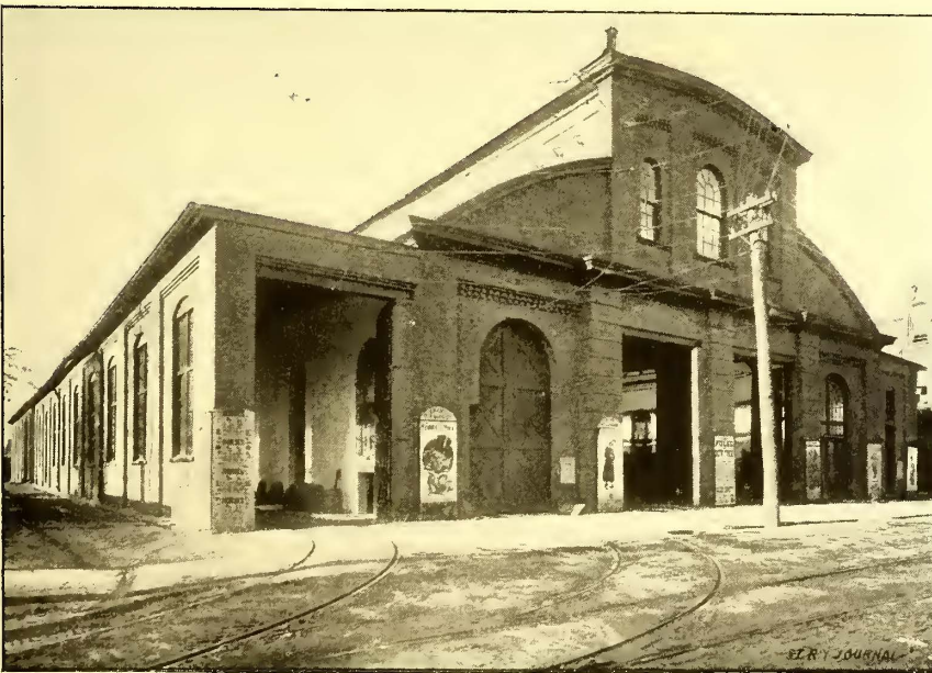
FIG. 6.—NORTHAMPTON STREET CAR HOUSE—WILKESBARRE & WYOMING VALLEY TRACTION CO.
