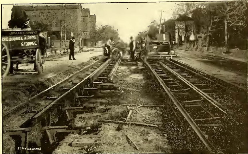
FIG. 8.—CABLE CONSTRUCTION ON COLUMBIA RAILROAD, SHOWING PORTABLE TOOL BOXES EMPLOYED.
