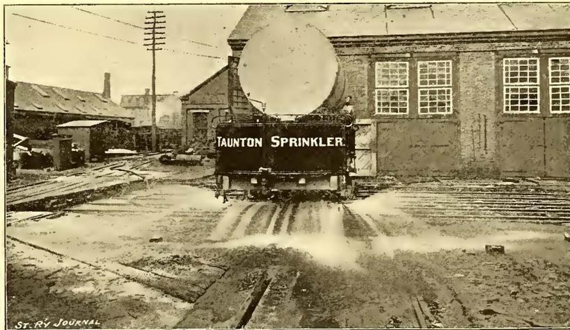
FIG. 2.—SPRINKLER WITH 40 FOOT SPREAD.
