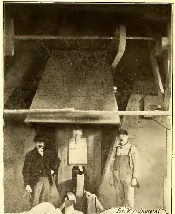
FIG. 6.—CLEANING WHEELS BY SAND BLAST.
