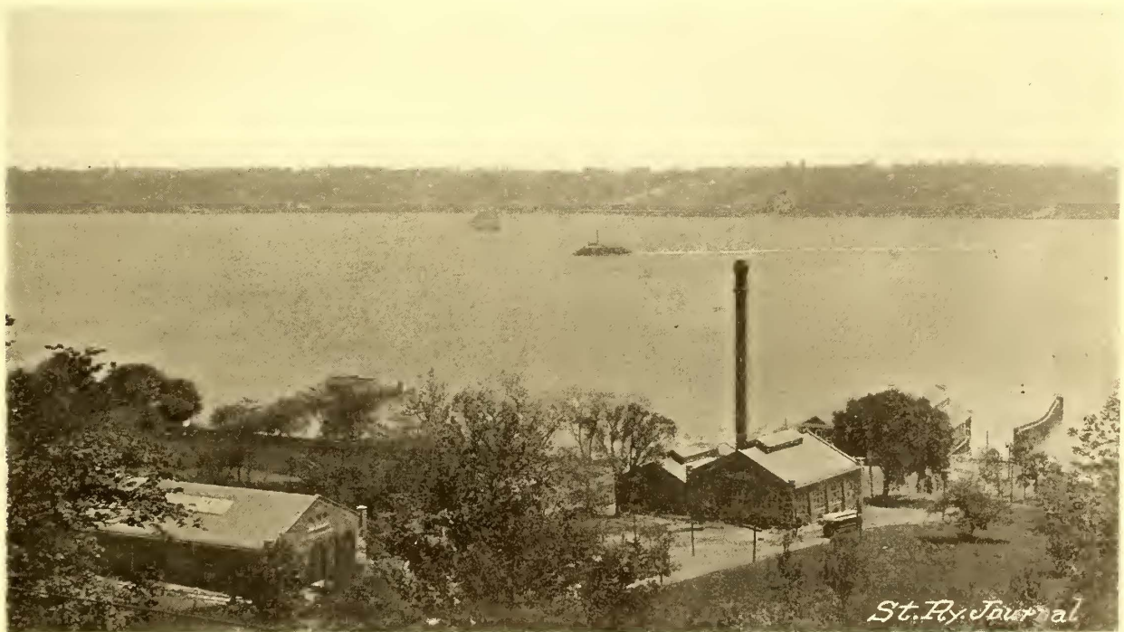
FIG. 1.—VIEW OF POWER STATION, CAR HOUSE AND UPPER END OF NEW YORK CITY FROM THE SWITCHBACK.
