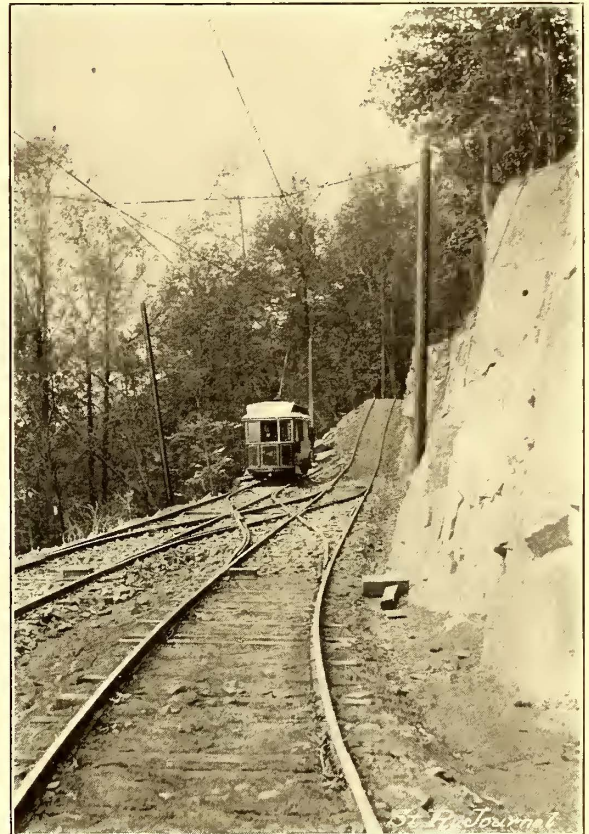
FIG. 13.—VIEW OF CAR ON SWITCHBACK, SHOWING SAFETY GRADE.
