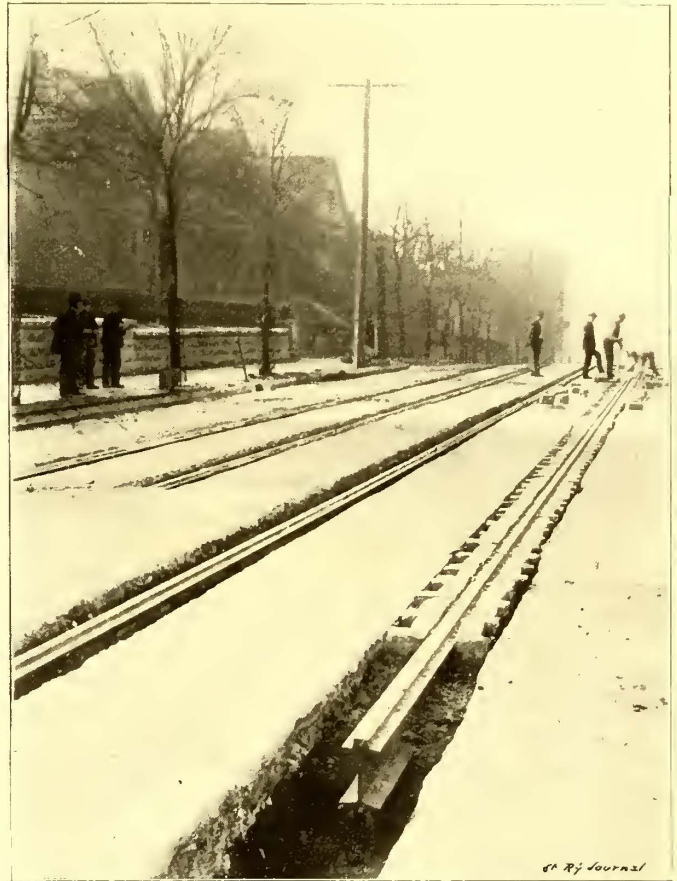
FIG. 7.—TRACK CONSTRUCTION ON THE WYANDOTTE STREET LINE
