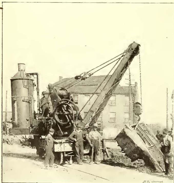
FIG. 3.—DERRICK FOR REMOVING DISCARDED CABLE CONDUIT
