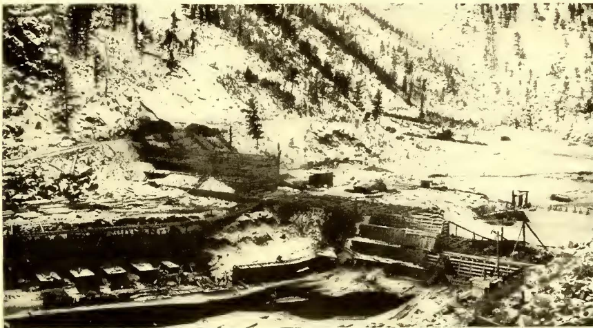
FIG. 2.—DAM LOOKING DOWN STREAM
