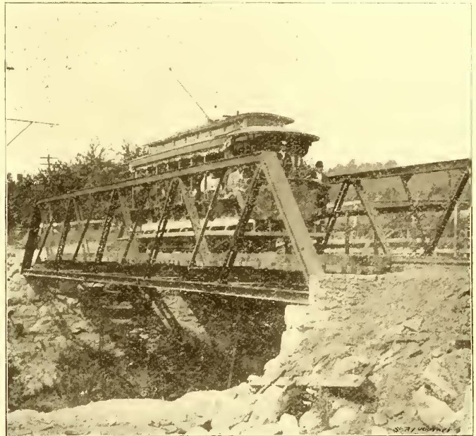
35 FT. GIRDER BRIDGE OVER ROBERTS CREEK
