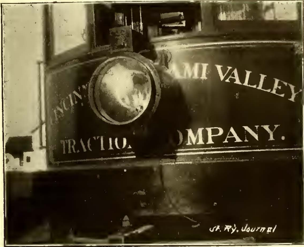
FIG. 4.—ELECTRIC ARC HEAD LIGHT.
