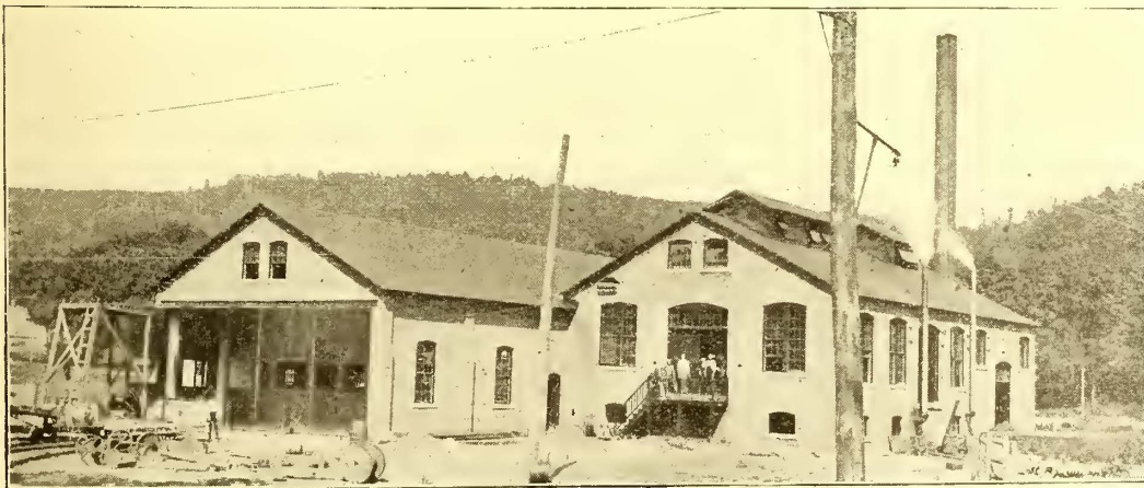
POWER STATION AND CAR HOUSE
