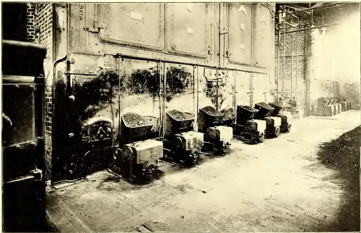
FIG. 1.—INTERIOR OF BOILER ROOM, SHOWING STOKERS—CINCINNATI
