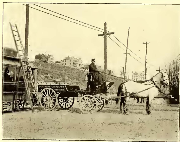
LADDER REMOVED FROM WAGON AND ERECTED NEAR CAR
