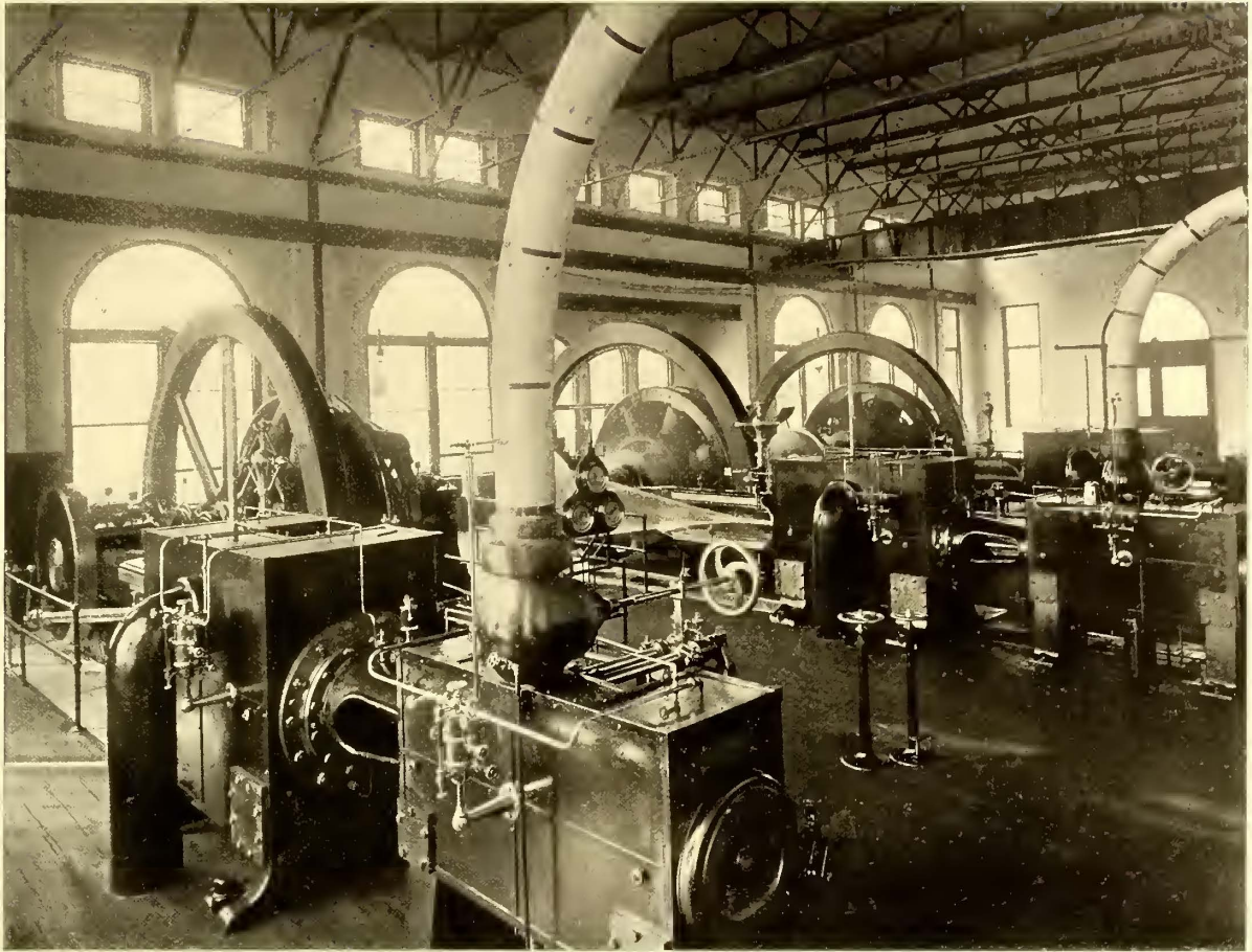
FIG. 13.—ENGINES—HOLYOKE POWER STATION
