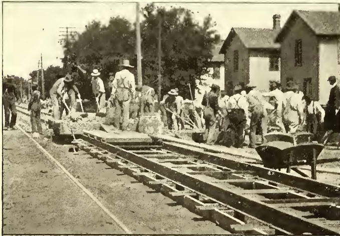
VIEW SHOWING BEAM FORMS IN POSITION
