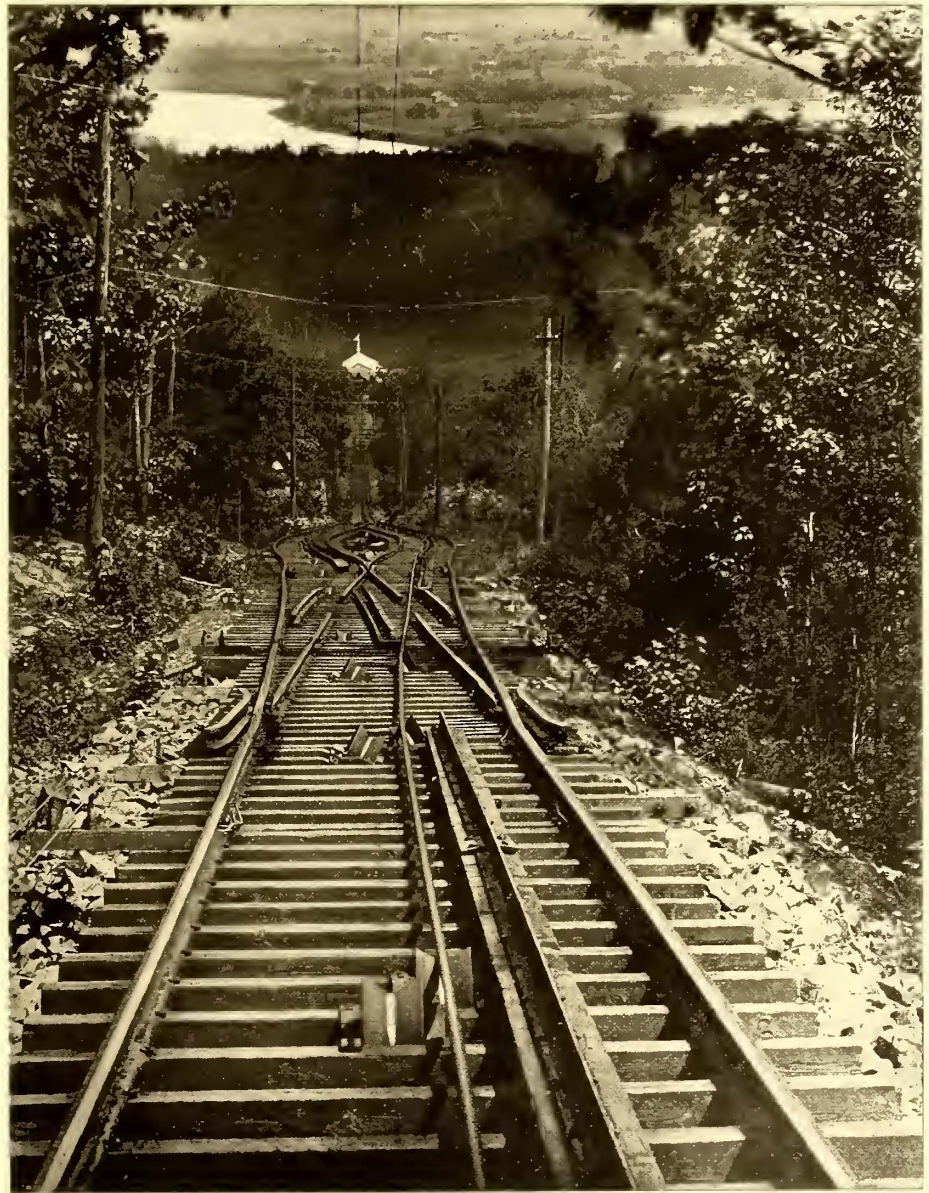
FIG. 16.—TURN-OUT, SHOWING ARRANGEMENT OF RAILS ALLOWING CAR TO PASS OVER CABLE OF OPPOSITE CAR
