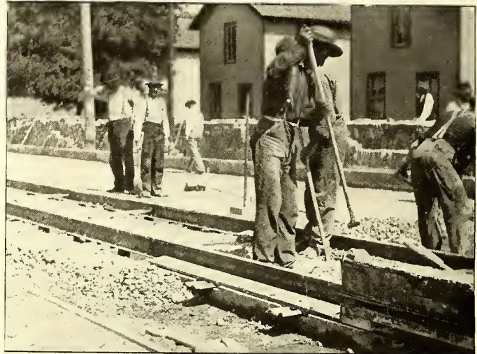
TAMPING PAVING CONCRETE UNDER TIES
