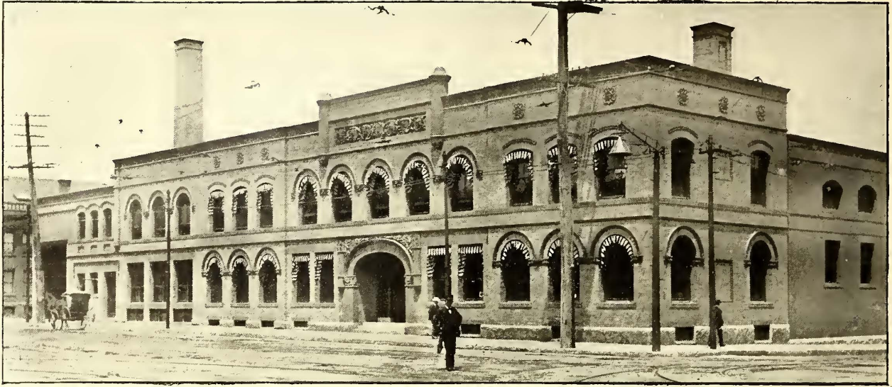
FIG. 5.—EXTERIOR OF CAR HOUSE—SPRINGFIELD
