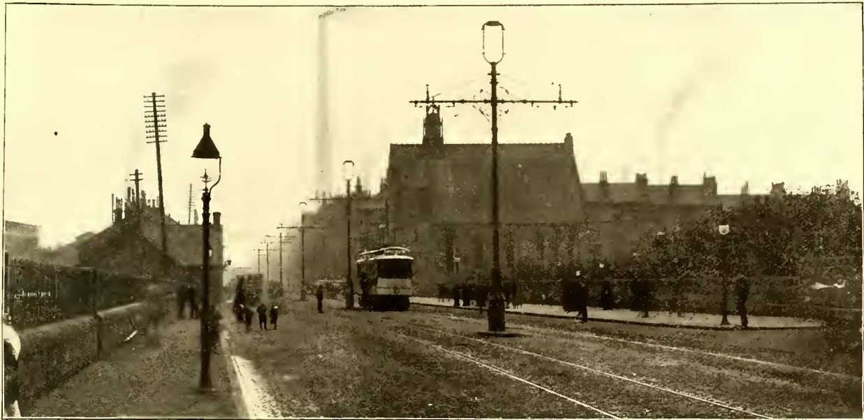
CENTER POLE CONSTRUCTION ON SPRINGBURN ROAD, GLASGOW
