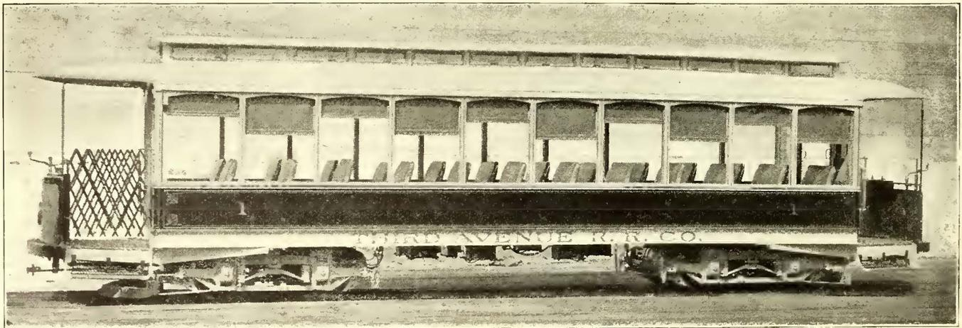
FIG. 9.—SIDE VIEW OF CAR, WHEN OPEN
