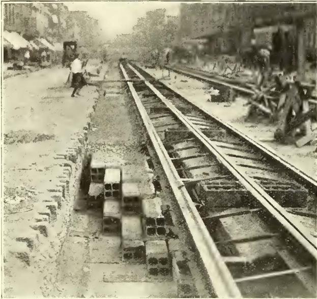
COVERING THE PIPES WITH CONCRETE
