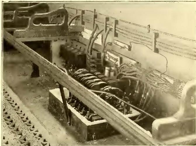
REVERSER AND RELAYS—MULTIPLE UNIT SYSTEM
