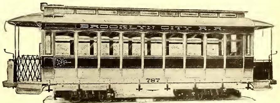
FIG. 2.—CONVERTIBLE CAR USED CLOSED
