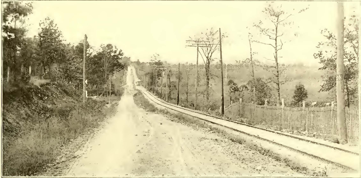
VIEW ON PONTIAC RAILWAY SHOWING TRACKS AT SIDE OF HIGHWAY
