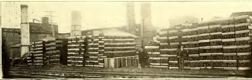
TERRA COTTA CONDUITS READY FOR SHIPMENT
