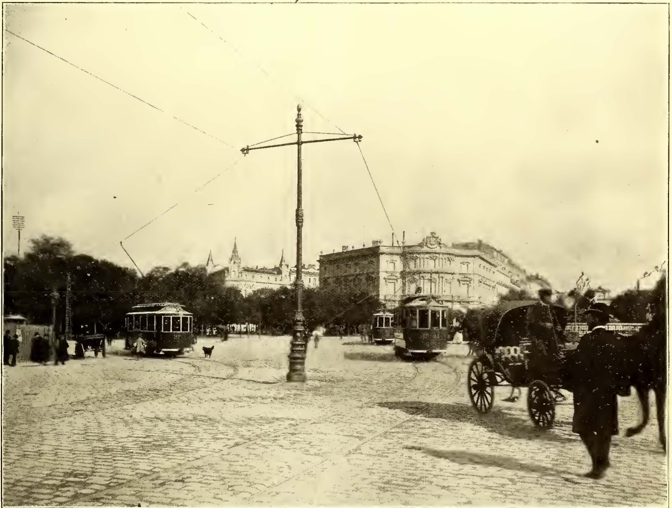
VIEW OF NEW ELECTRIC LINE AT MADRID
