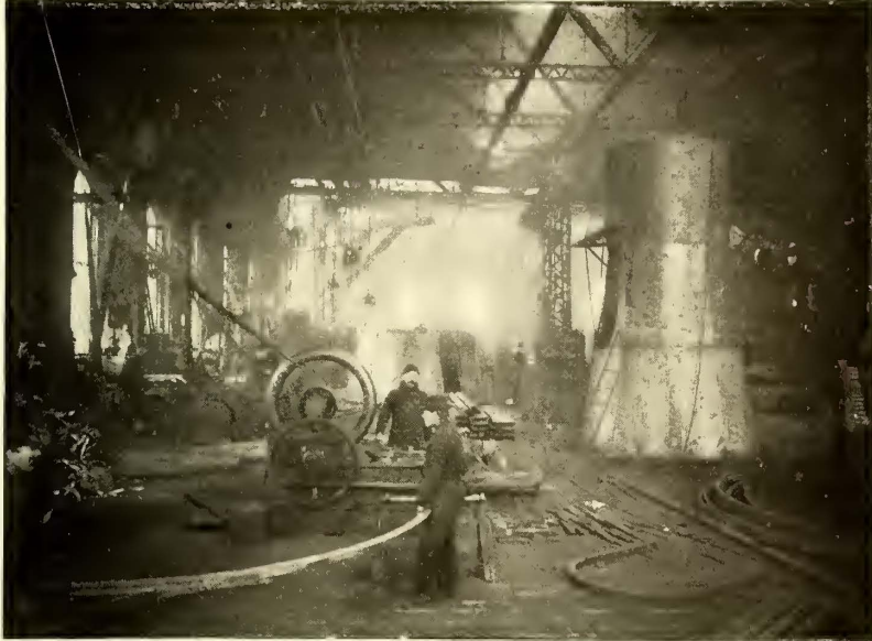
CONSTRUCTING A 200 FT. SELF-SUPPORTING STACK
