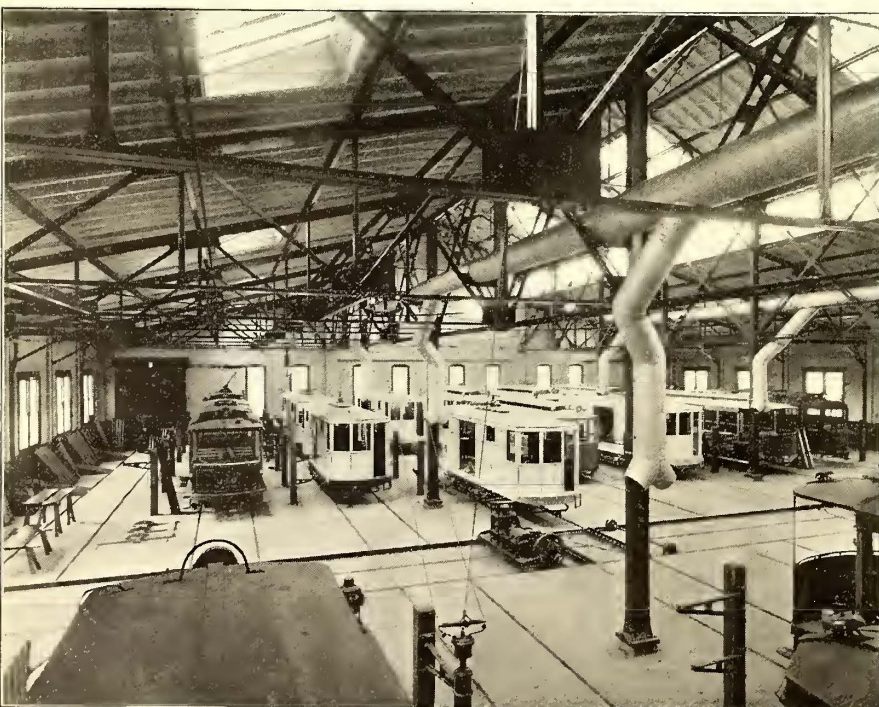
PAINT SHOP, SHOWING ELECTRIC TRANSFER TABLE, BRACKETS FOR SCAFFOLDING AND HEATING TUBES
