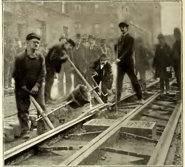
FIG. 4.—CASTING JOINT
