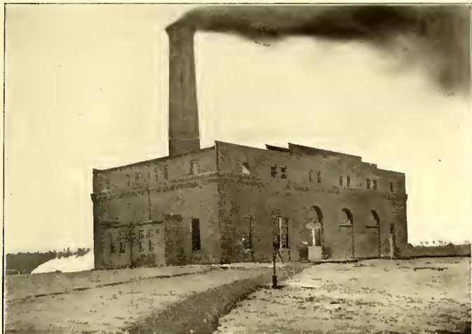
EXTERIOR OF POWER STATION
