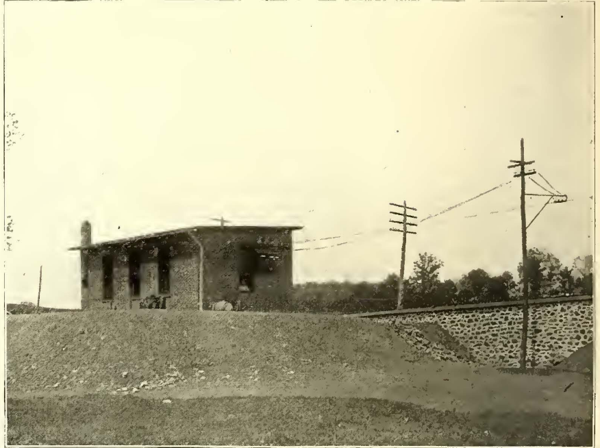
EXTERIOR OF ROTARY CONVERTER SUBSTATION
