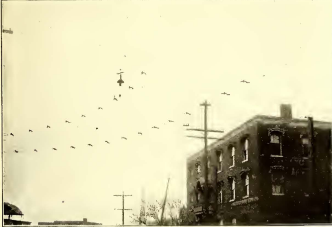
CURVE CONSTRUCTION WITH FIG. 8 TROLLEY WIRE
