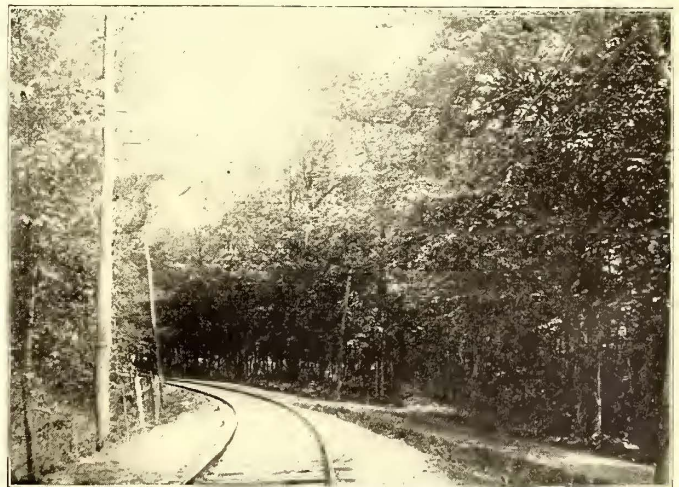
CONSTRUCTION NEAR WILMINGTON
