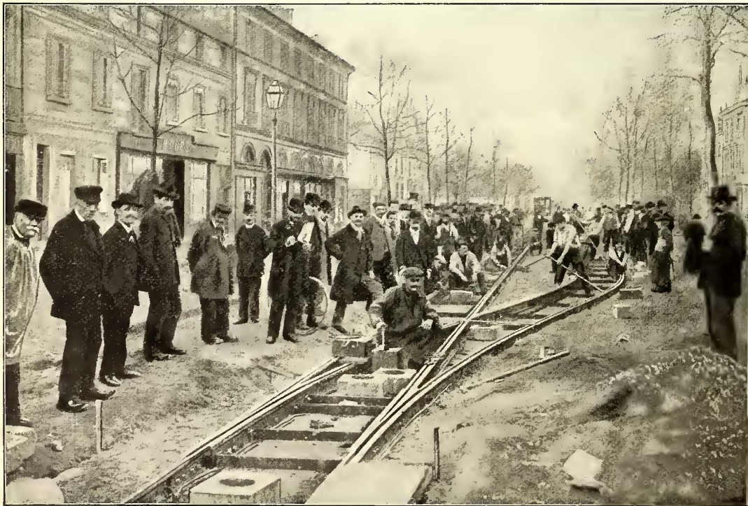
LAYING THE TRACK
