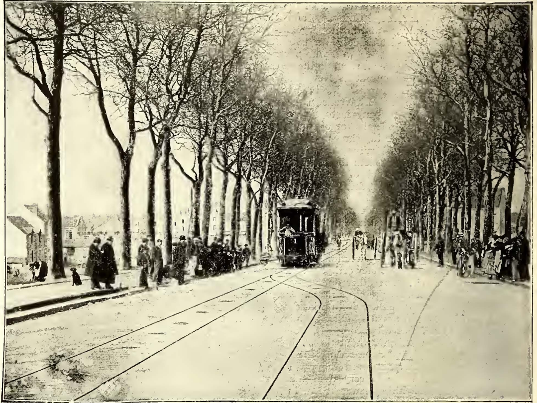
SECTION OF COMPLETED TRACK
