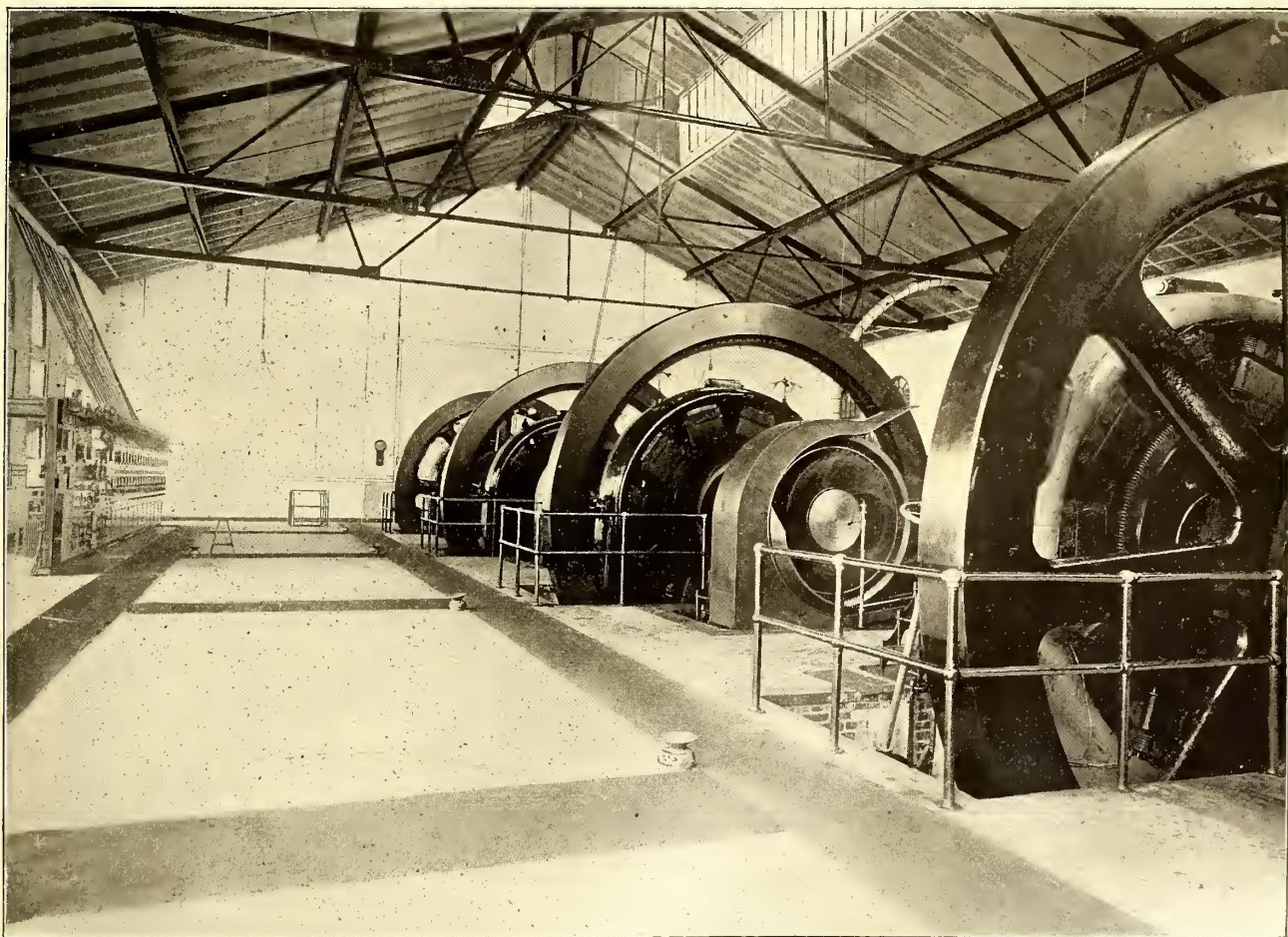
VIEW IN POWER STATION OF UNITED TRACTION COMPANY, PITTSBURGH
