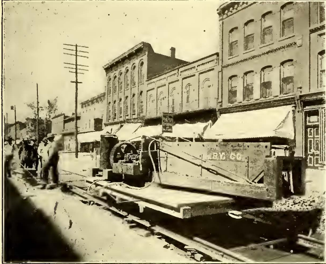
VIEW OF BALLAST CAR
