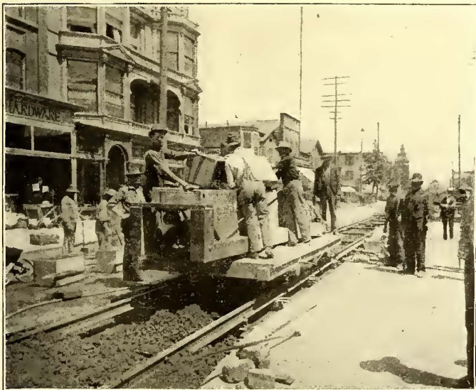
DUMPING BALLAST FROM CAR
