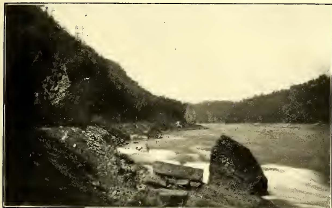
GIANT ROCK ON LEFT, DEVIL'S HOLE RAPIDS ON RIGHT. VIEW TAKEN DURING CONSTRUCTION
