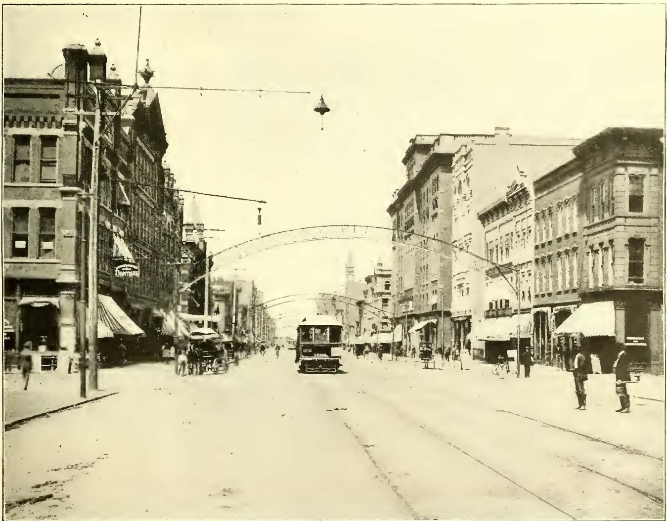
VIEW ON HIGH STREET, SHOWING METHOD OF ARCH ILLUMINATION
