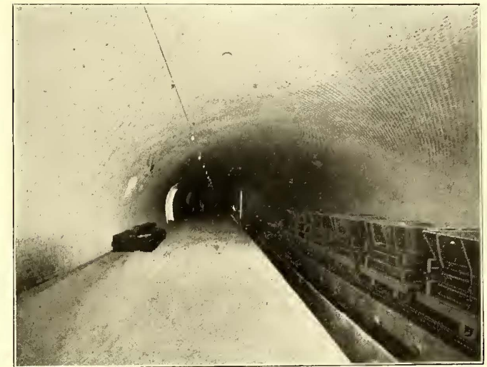
FIG. 12.—INTERIOR PLACE DE L'ETOILE STATION, TROCADERO BRANCH
