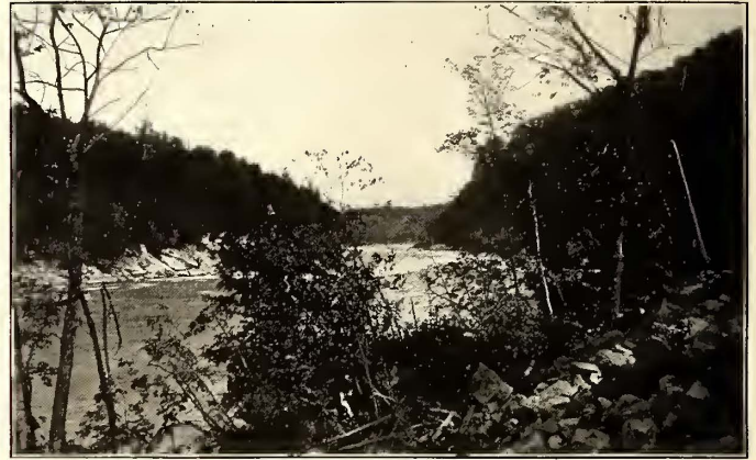
ONGIARA POINT, VIEW TAKEN DURING SURVEY
