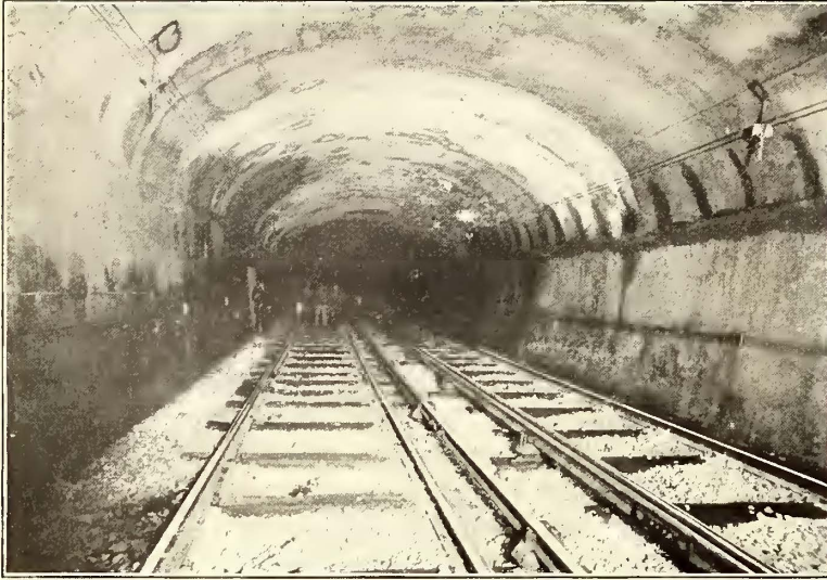
FIG. 15.—VIEW IN TUNNEL PORTE MAILLOT—VINCENNES LINE
