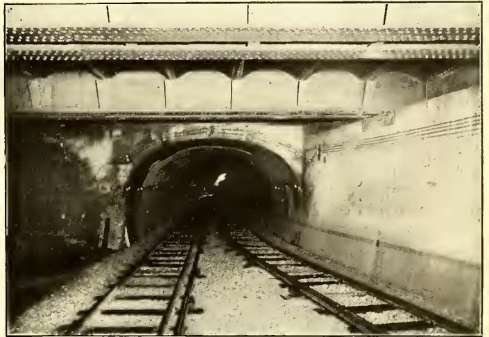
FIG. 18.—TUNNEL AT LYON STATION
