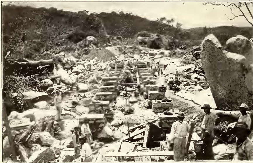
MASONRY FOUNDATION FOR MAIN FEEDER TUBE
