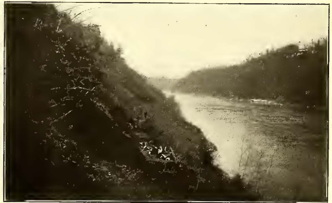
BEGINNING WORK ON TALUS NEAR LEWISTON
