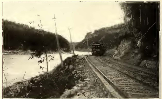
ONGIARA POINT, VIEW TAKEN AFTER COMPLETION OF ROAD
