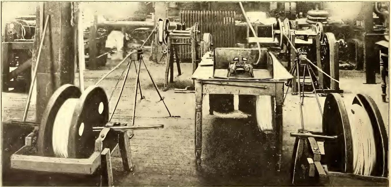
FIG. 9.—FIELD COIL WINDERS
