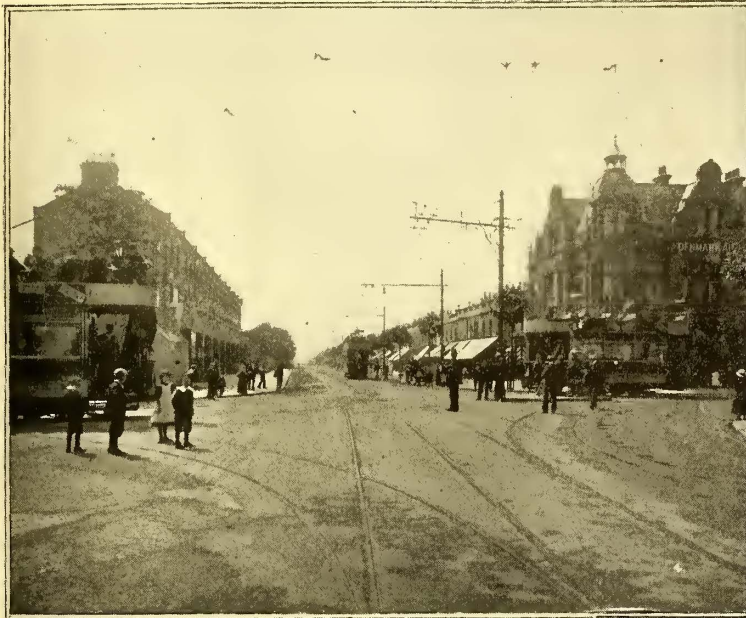
SIDE POLE CONSTRUCTION
