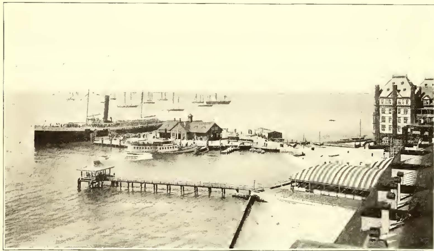
TERMINAL AT OLD POINT
