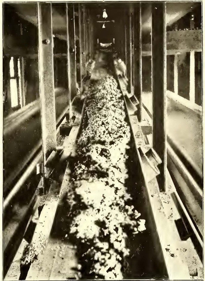
ASH CONVEYORS AT NINETY-SIXTH STREET STATION
