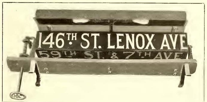
SIGN TIPPED TO SHOW LAMPS AND MECHANISM
