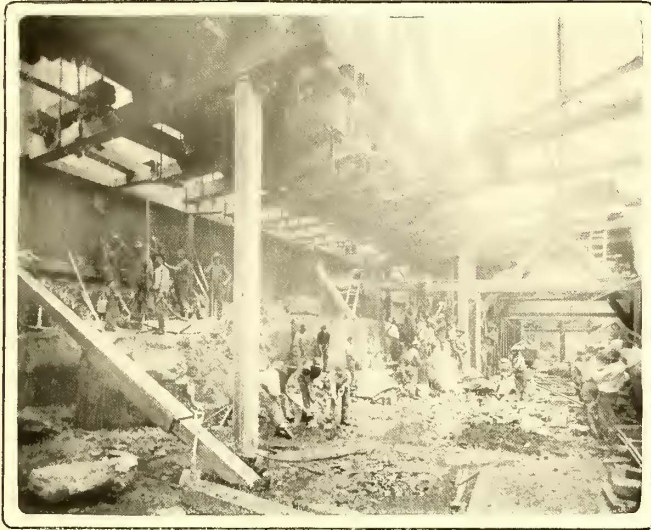
FIG. 9.—STREET RAILWAY TRACK ON TEMPORARY SUPPORTS
