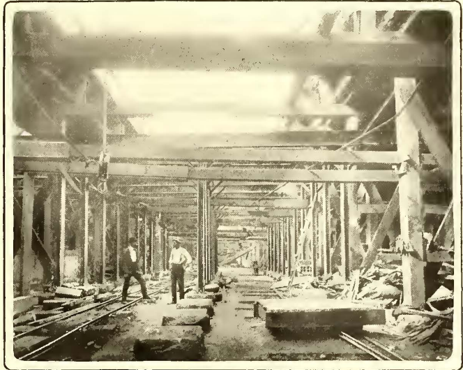
FIG. 10.—STRUCTURE IN MIDDLE OF STREET UNDER BOTH STREET RAILWAY TRACKS
