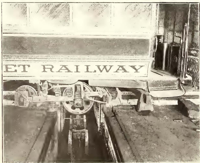
PITS FOR WHEEL RENEWAL
