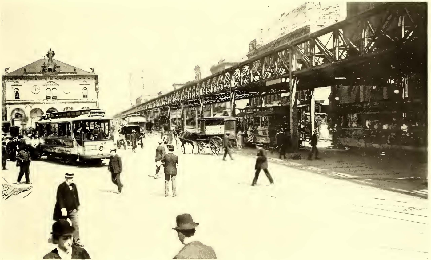
HERALD SQUARE, MANHATTAN, WHERE 1070 SURFACE CARS PASS IN AN HOUR
