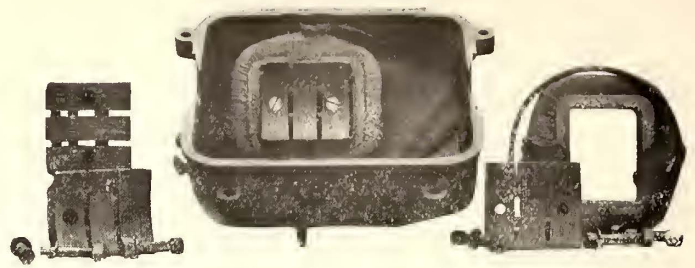
FIG. 4.—DETAILS OF POLE PIECES AND FIELDS
