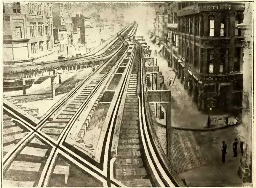
PROPOSED CONNECTION OF ELEVATED ROADS
