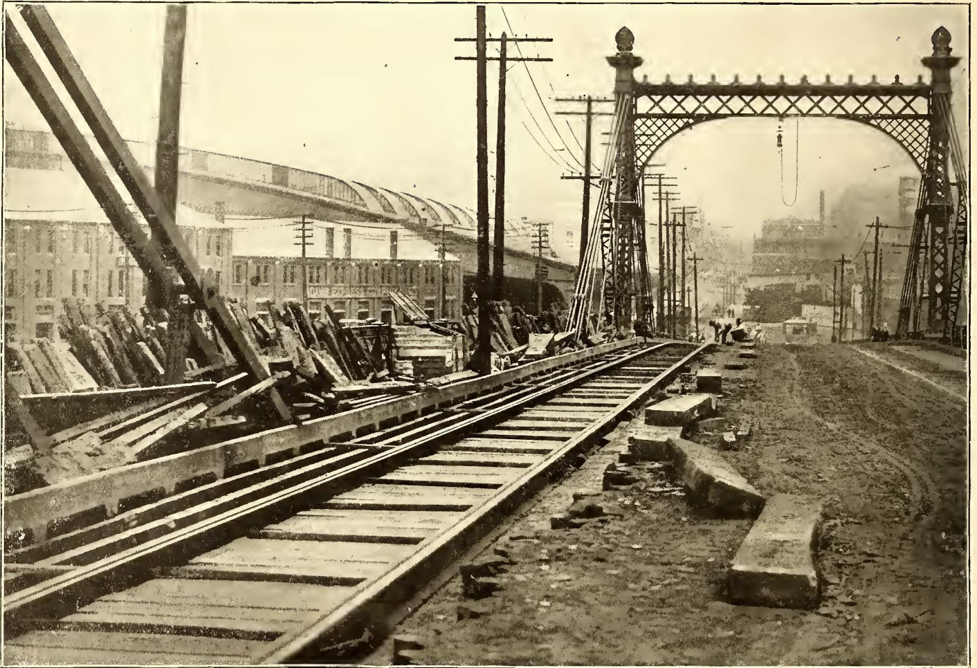
TRACK CONSTRUCTION ON 18TH STREET, ST. LOUIS
