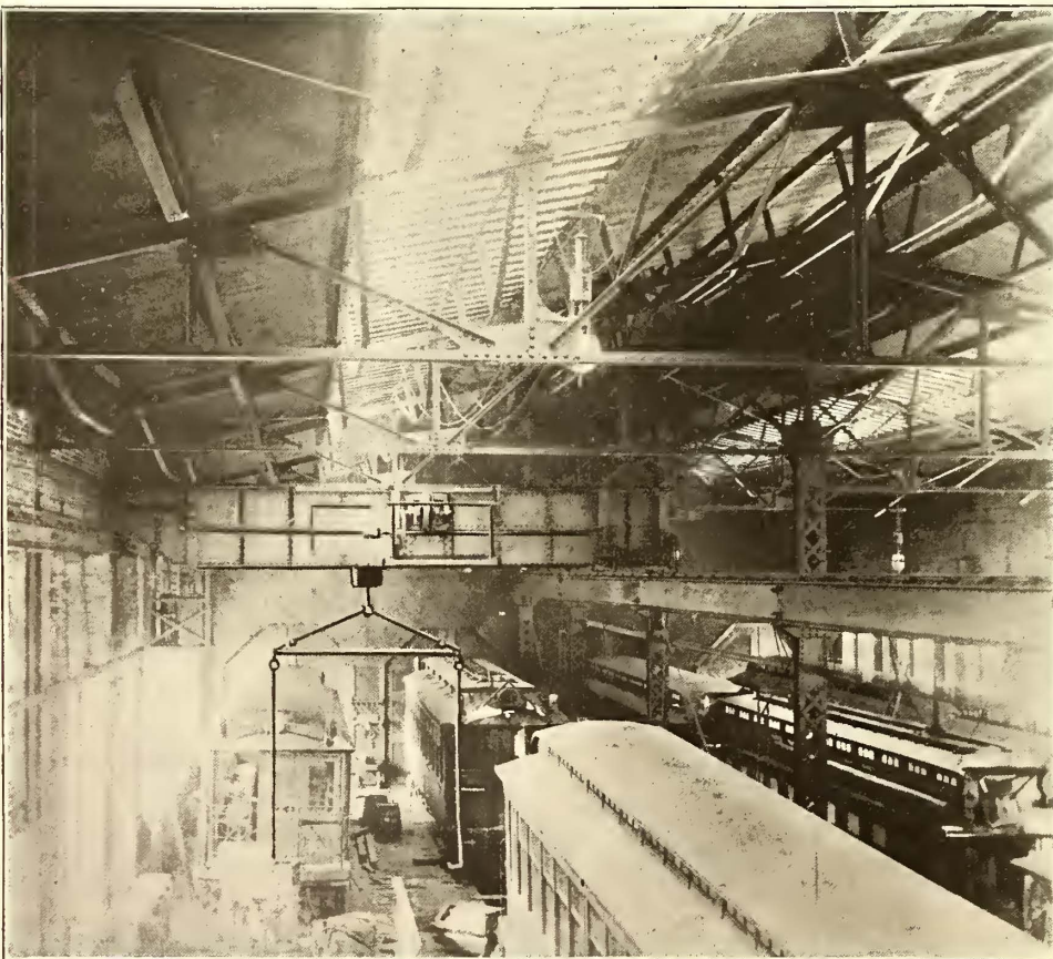
FIG. 6—LAKE ST. ELEVATED SHOPS. CRANE AND YOKE FOR LIFTING CAR BODIES
