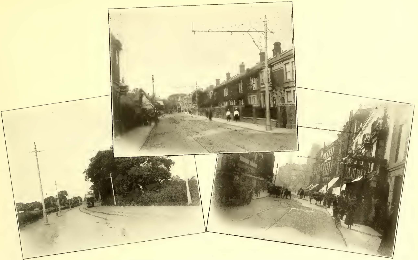
SOME TYPICAL OVERHEAD CONSTRUCTION, PORTSMOUTH
