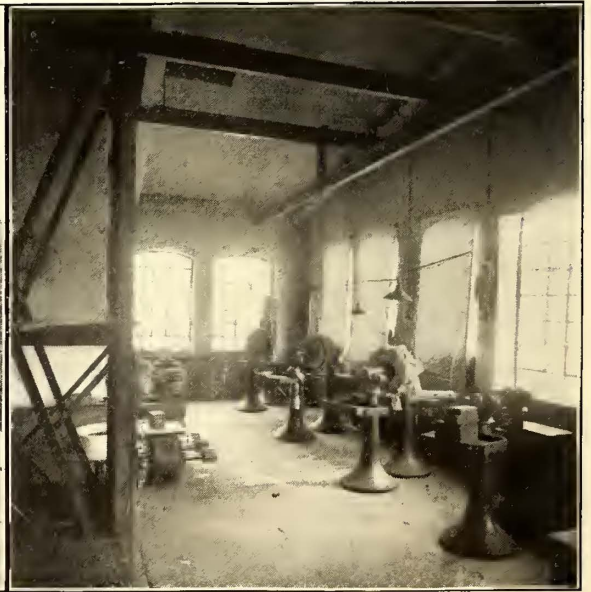
ARMATURE REPAIR ROOM
