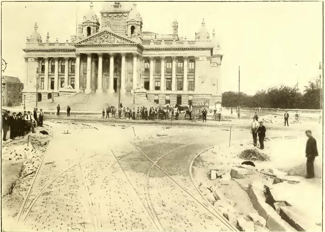
TRACK WORK IN FRONT OF TOWN HALL, PORTSMOUTH
