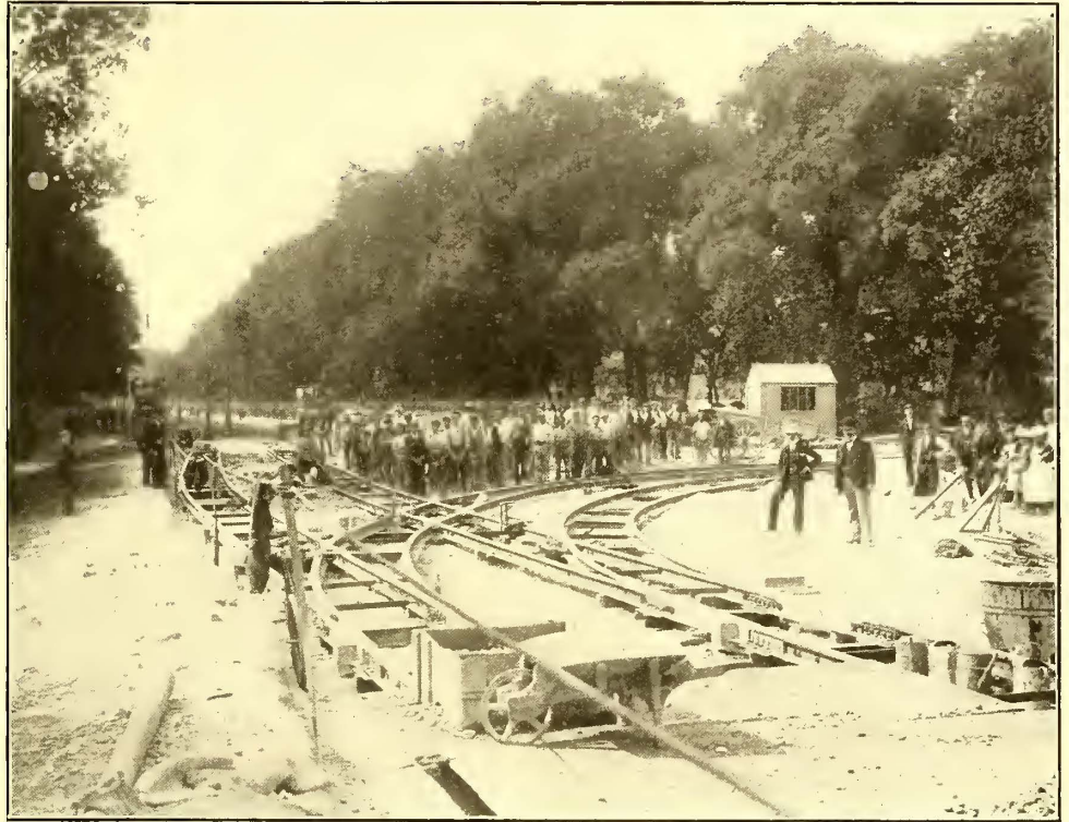
A FINE PIECE OF SPECIAL WORK, BRIGHTON
