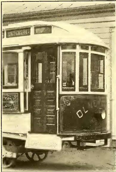
FIG. 4.—ENTIRELY ENCLOSED VESTIBULE, MODIFIED STEAM TYPE
