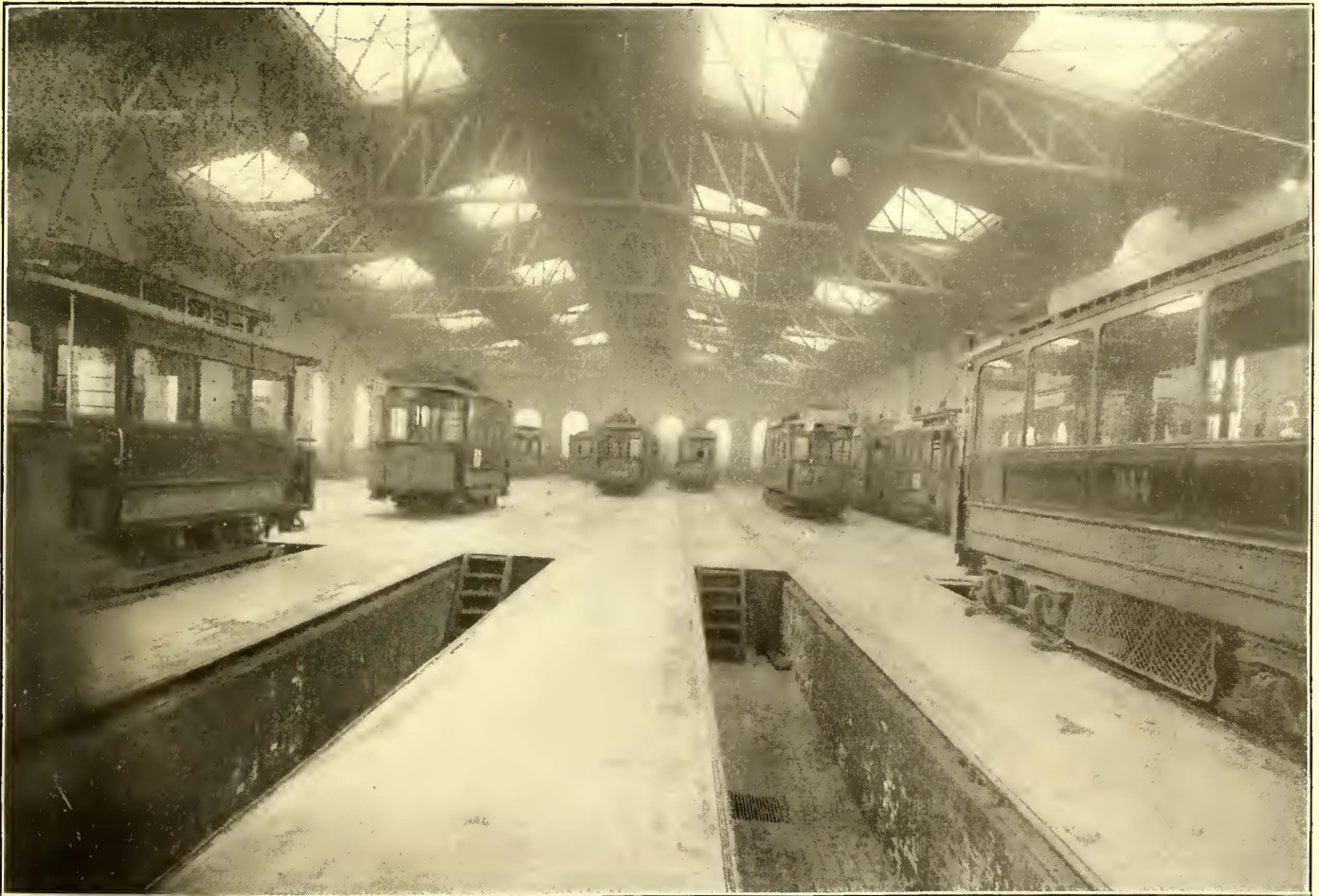
LEHMWEG CAR HOUSE
