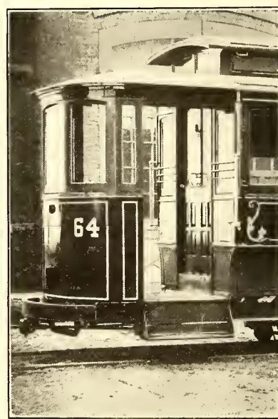
FIG. 3.—OPEN VESTIBULE WITH SASH SET AT SIDE
