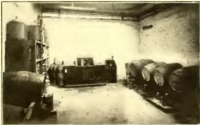
OIL AND PAINT ROOM
