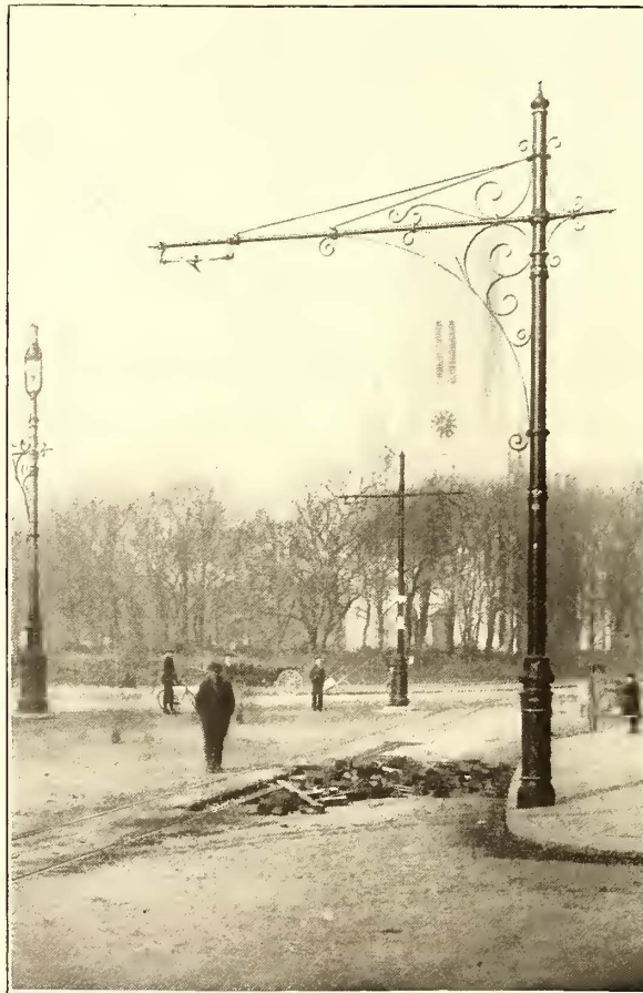
SPAN AND BRACKET POLES USED IN BRIGHTON
