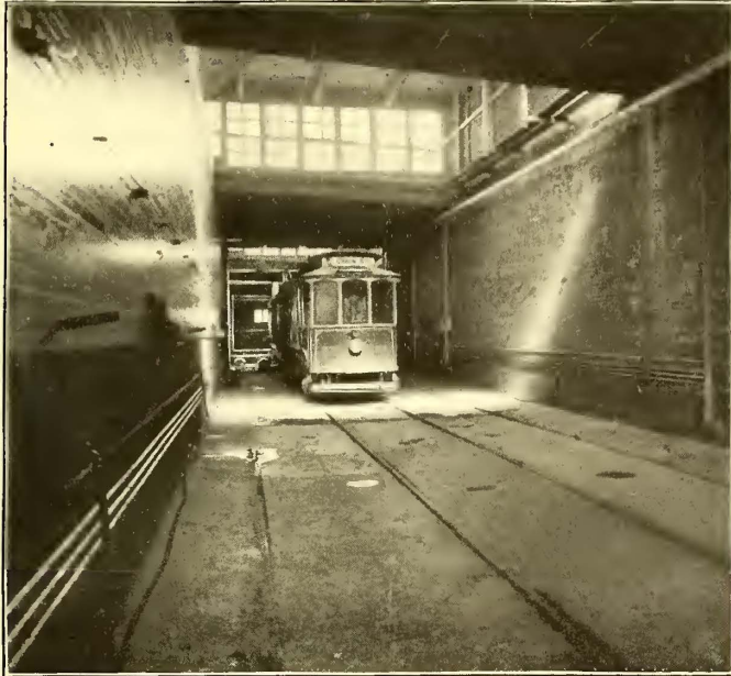
WASH ROOM—GATES LANE CAR HOUSE
