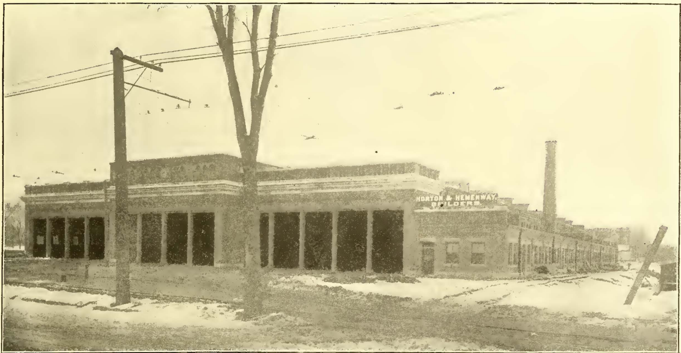
EXTERIOR OF CAR HOUSE
