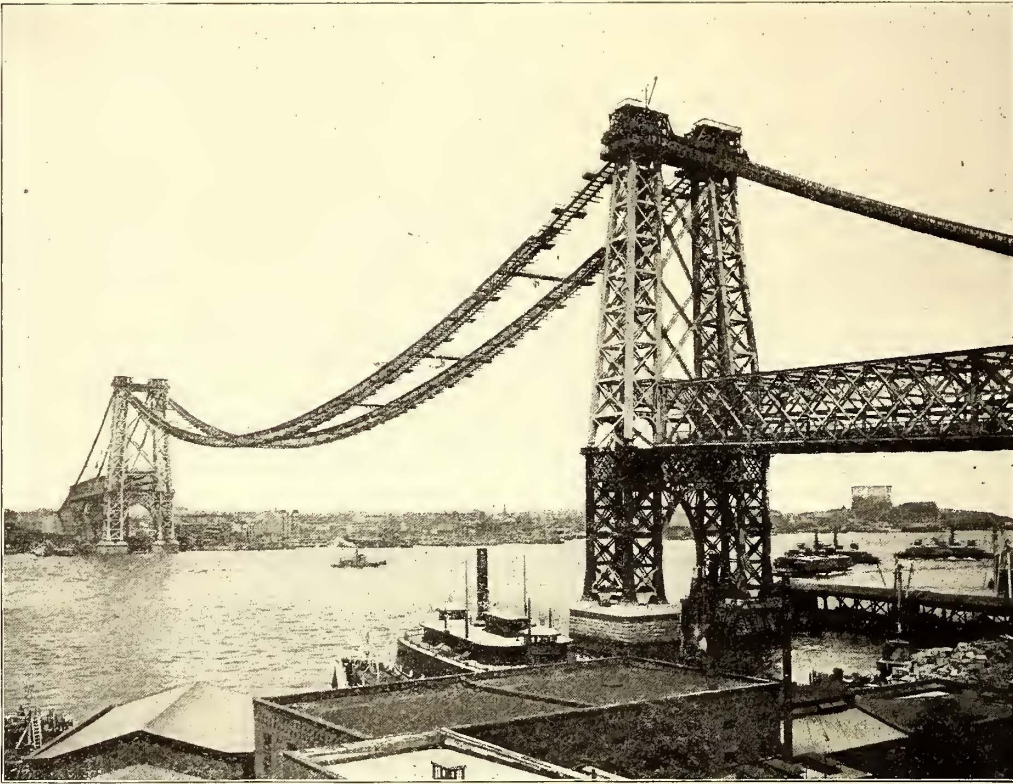
NEW EAST RIVER BRIDGE
