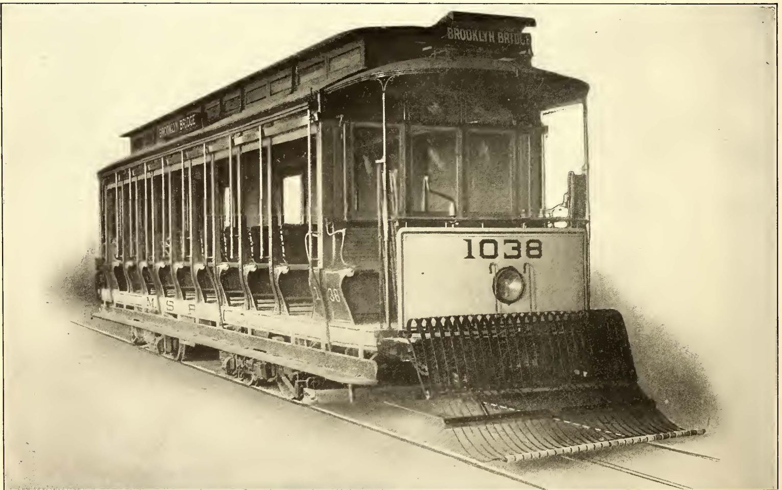
FRONT VIEW OF CAR EQUIPPED WITH MODEL “A” CAR FENDER
