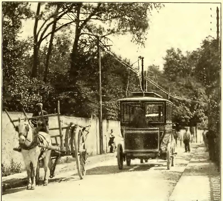
AUTO-TROLLEY LINE ON ROAD TOO NARROW FOR STREET RAILWAY
