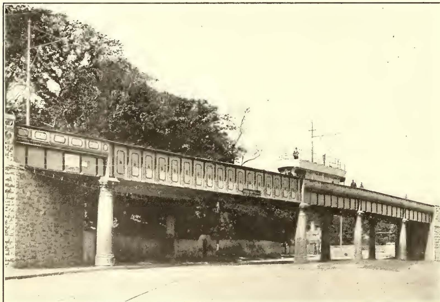
STEEL BRIDGE CARRYING TRAMWAY INTO RAILWAY STATION AT HOWTH
