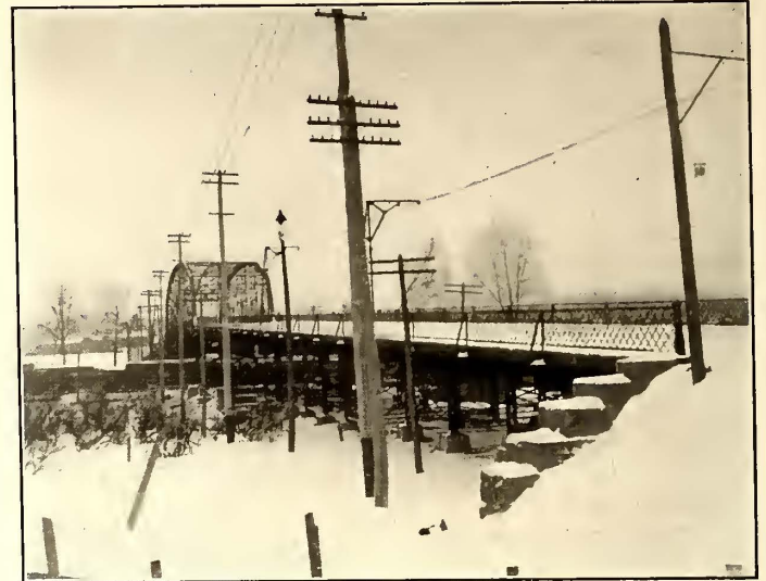
VIADUCT CROSSING STEAM RAILROAD
