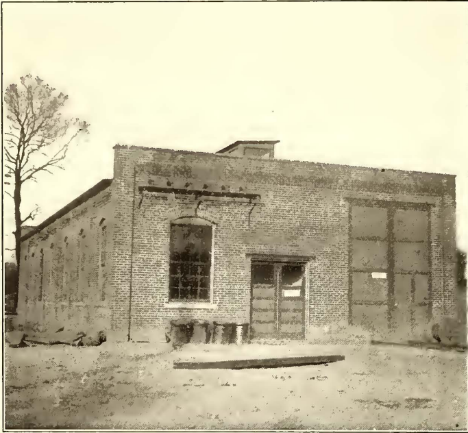
COMBINED SUB-STATION AND CAR HOUSE
