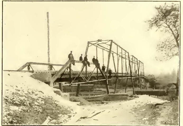
LONG BRIDGE CROSSING STEAM RAILROAD TRACKS
