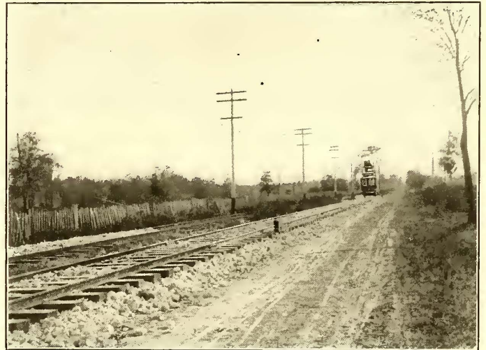
CONSTRUCTING THE OVERHEAD LINE WITH OLD CAR
