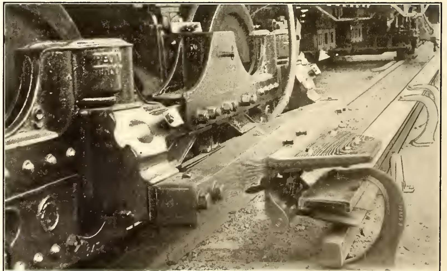
CONTACT SHOE ENTERING PROTECTED THIRD RAIL
