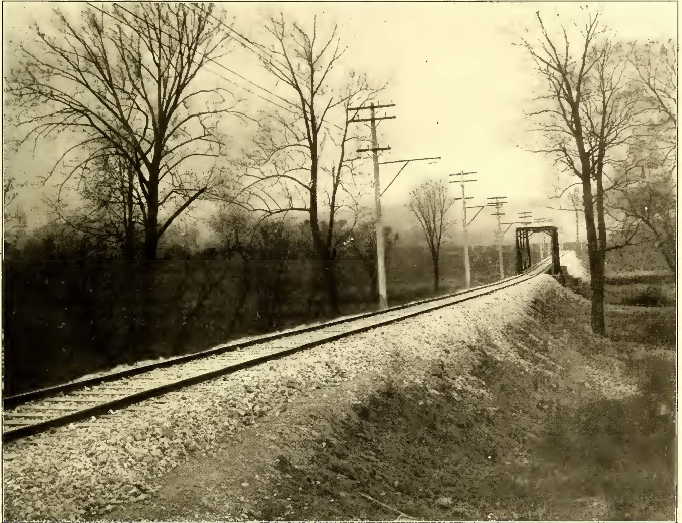
A GOOD EXAMPLE OF THE TRACK CONSTRUCTION
