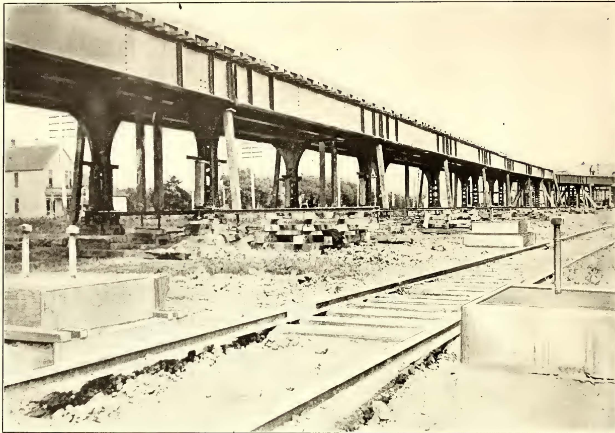
METHOD OF MOVING STRUCTURE
