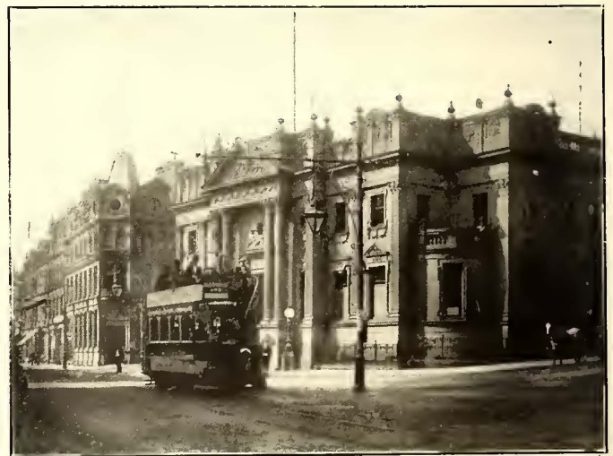
FIG. 11.—VIEW SHOWING OVERHEAD CONSTRUCTION
