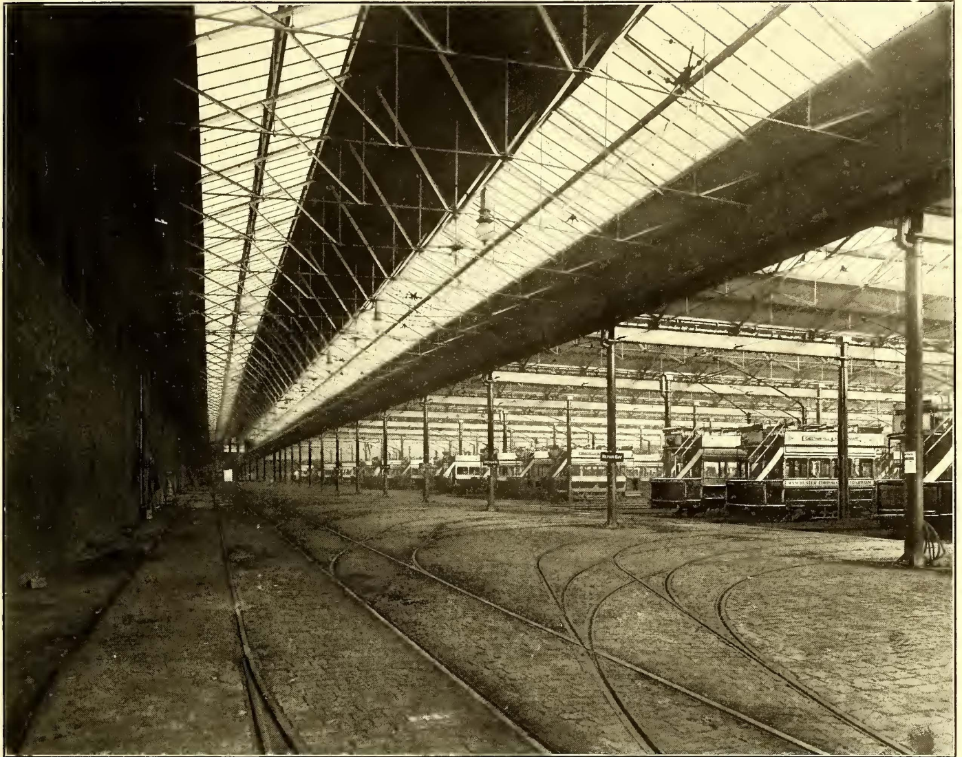
FIG. 2.—INTERIOR OF NEW QUEEN'S ROAD CAR HOUSE
