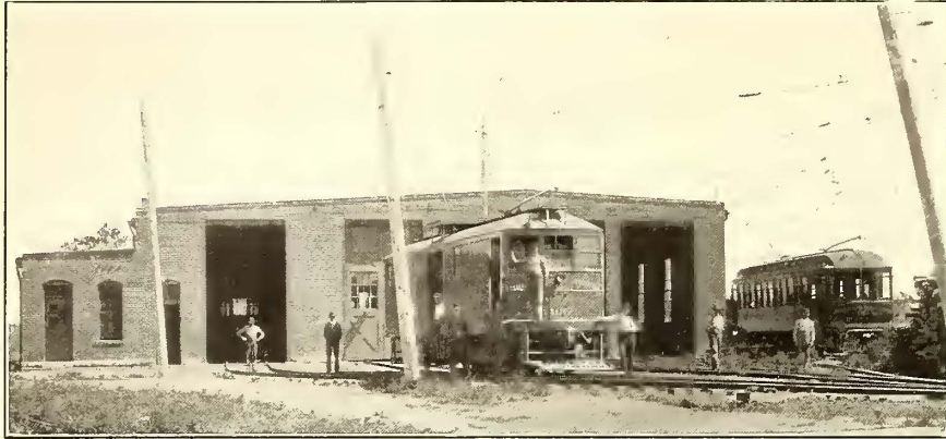
CAR SHEDS, SHOWING FREIGHT CAR WITH TOP PLATFORM FOR LINE REPAIR WORK
