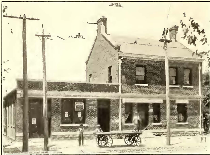
SUB-STATION, FREIGHT HOUSE AND AGENT'S RESIDENCE
