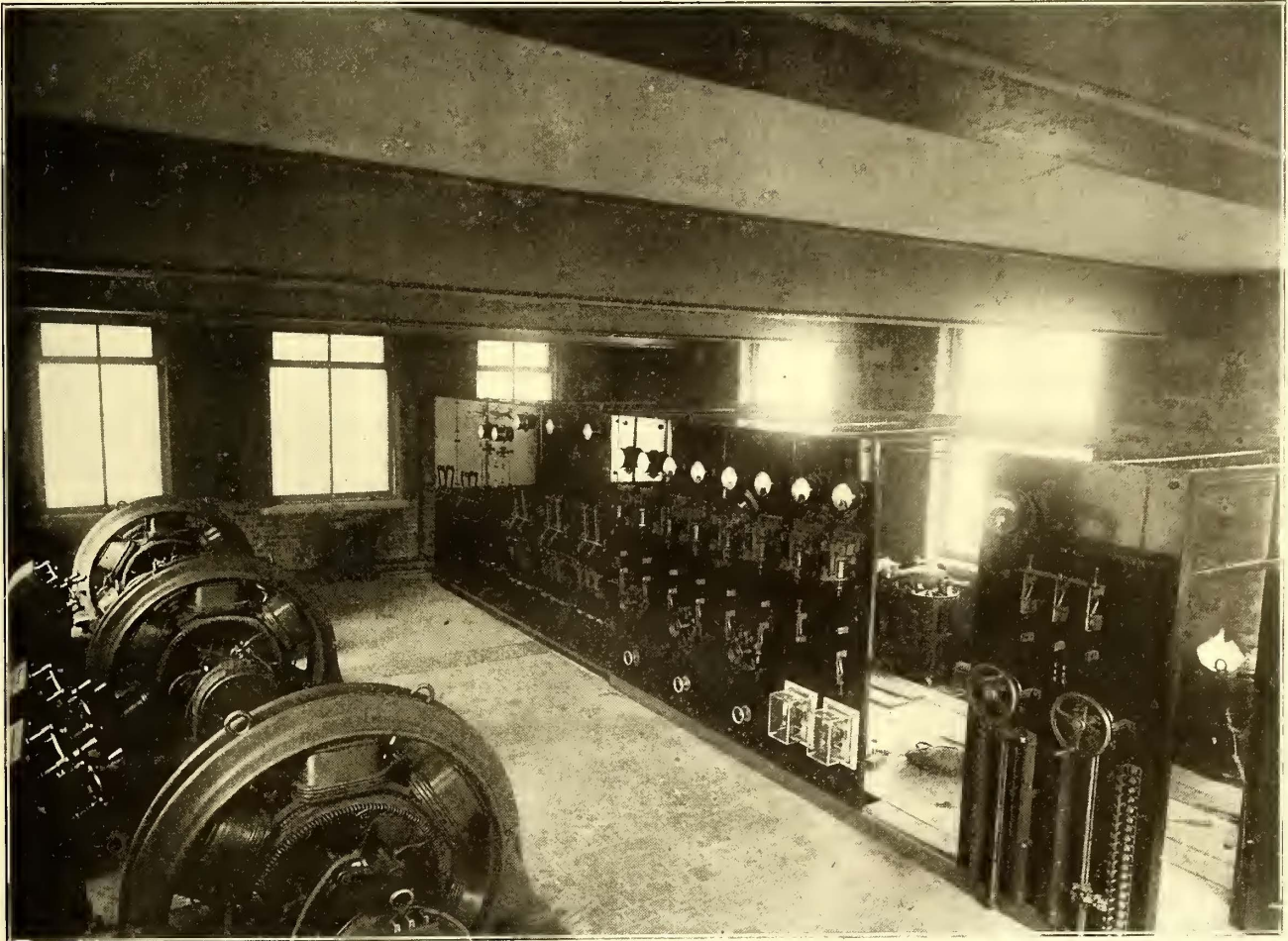
FIG. 9.—SUB-STATION AT HEBDEN BRIDGE
