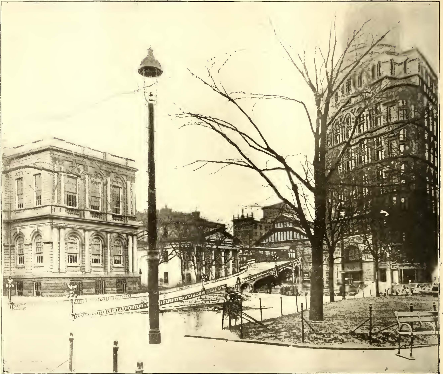
ENTRANCE TO BROOKLYN BRIDGE, SHOWING PROPOSED INCLINED APPROACH TO ELEVATED LINES FROM CITY HALL PARK
