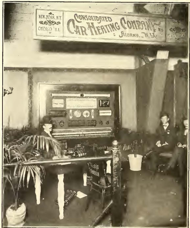
EXHIBIT OF THE CONSOLIDATED CAR HEATING COMPANY
