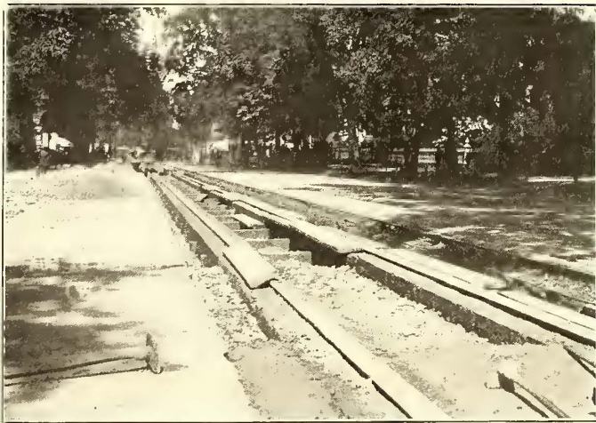
VIEWS OF HARTFORD TRACK CONSTRUCTION, SHOWING METHOD OF LAYING RAILS IN CONCRETE
