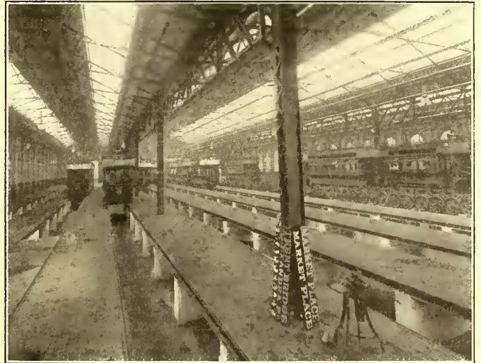
INTERIOR OF TRENT BRIDGE CAR HOUSE
