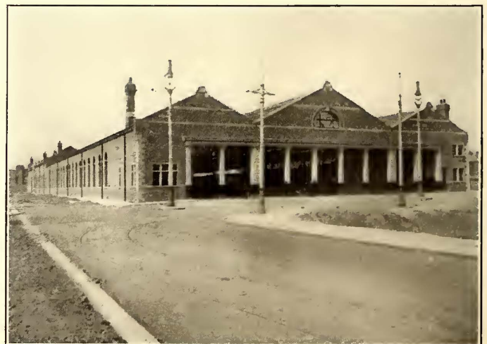
EXTERIOR OF TRENT BRIDGE CAR HOUSE
