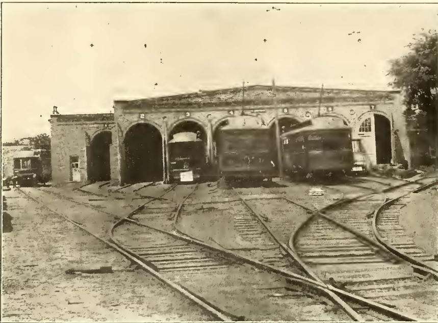
CAR SHEDS AND REPAIR SHOPS AT SYLVANIA
