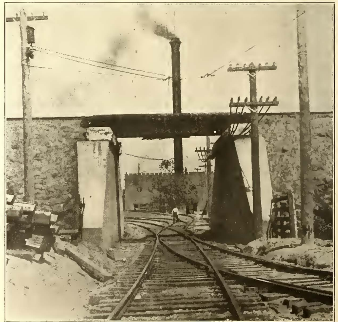
CROSSING UNDER STEAM RAILROAD
