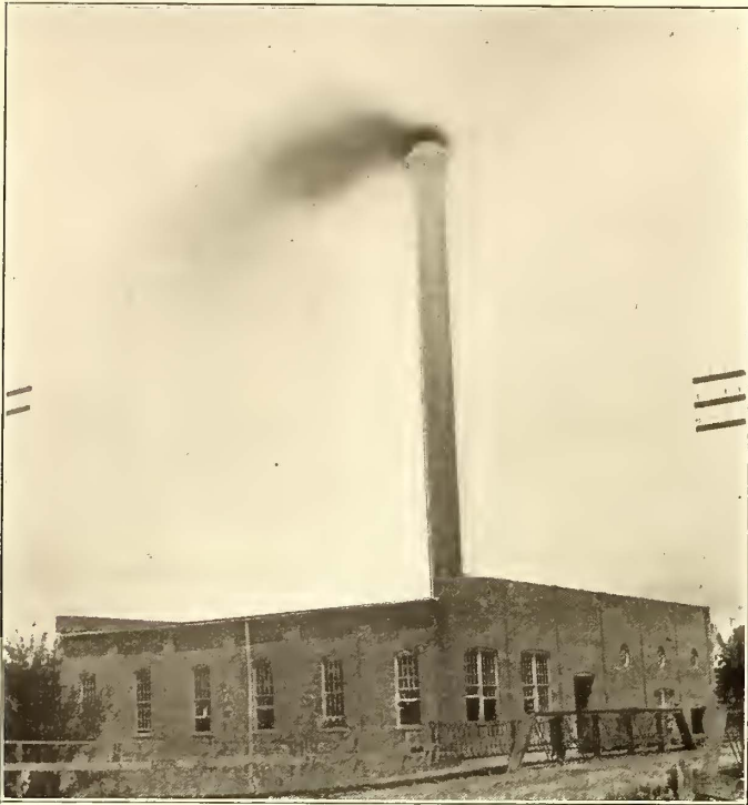
MAIN POWER HOUSE AT SYLVANIA
