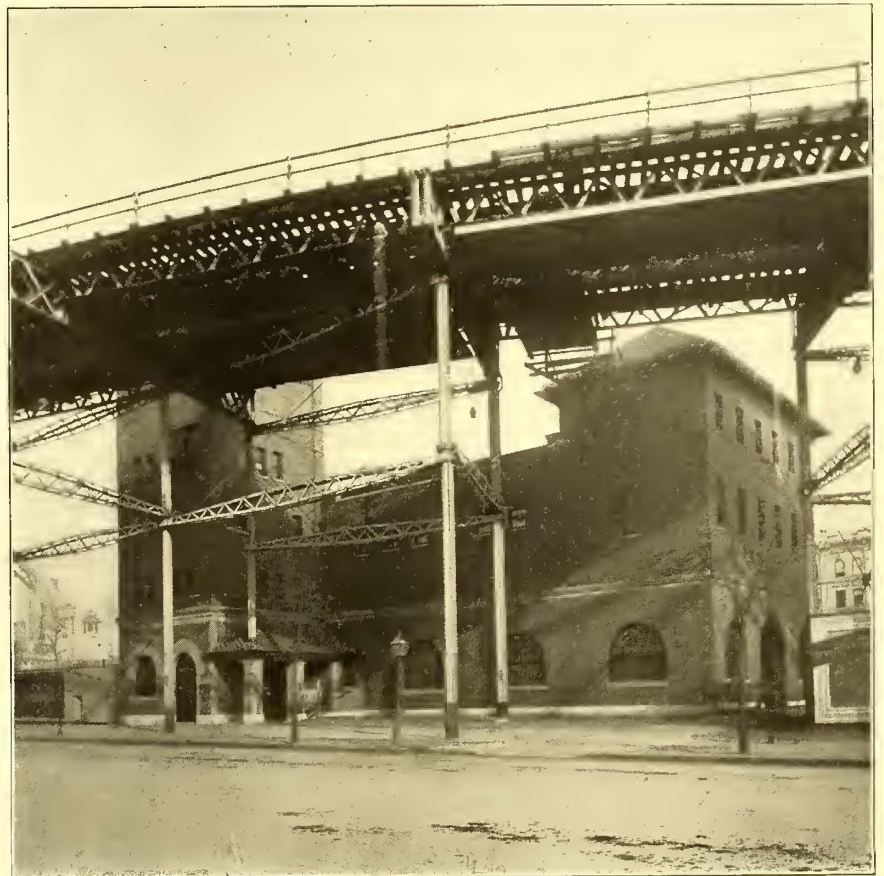
FIG. 2.—COMBINED PASSENGER AND ROTARY SUB-STATION AT 110TH STREET LOOP, FACING CENTRAL PARK
