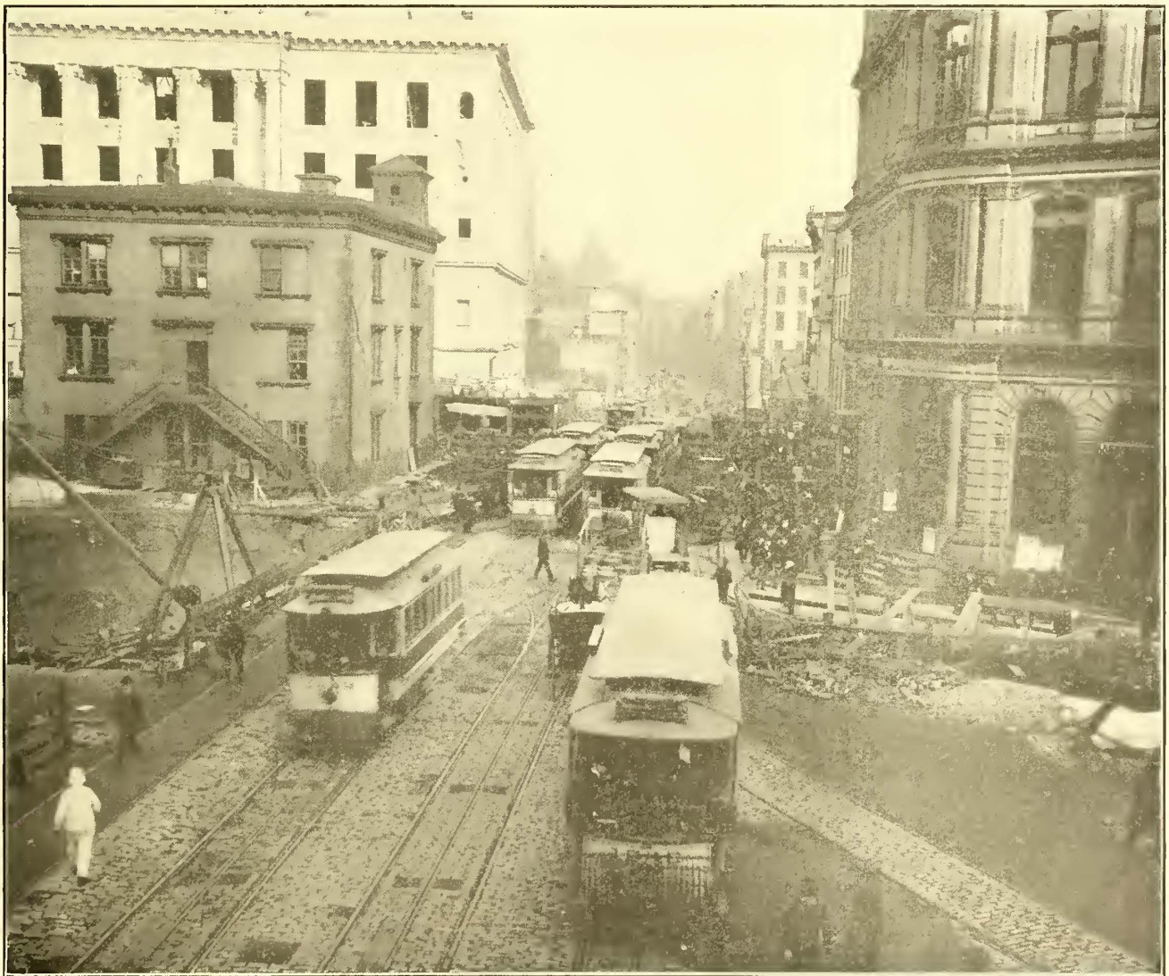
OBSTRUCTIONS ON CENTER STREET CAUSED BY SUBWAY EXCAVATIONS
