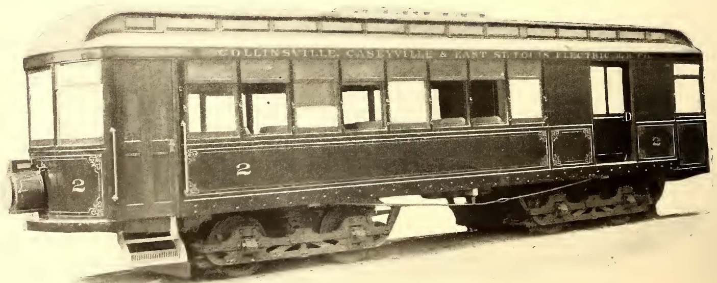
32 FT. VESTIBULED BAGGAGE AND PASSENGER CAR FOR INTERURBAN TRAFFIC
