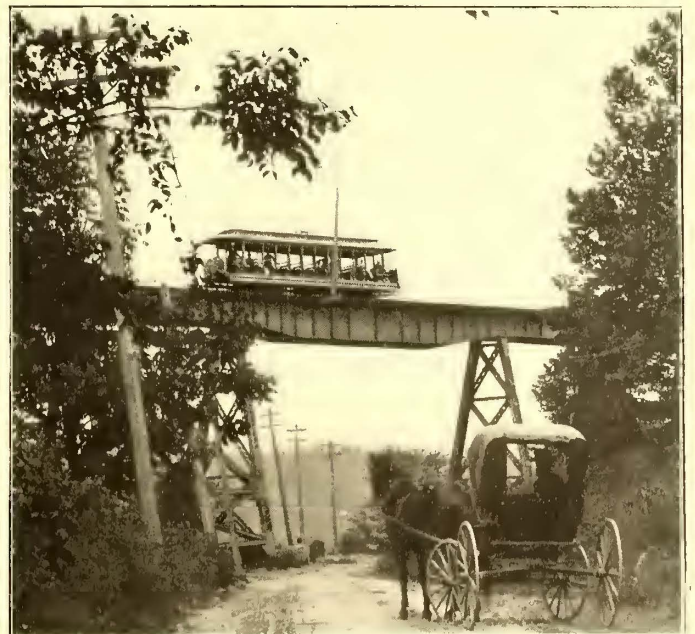
TYPICAL BRIDGE OVER HIGHWAY CROSSING
