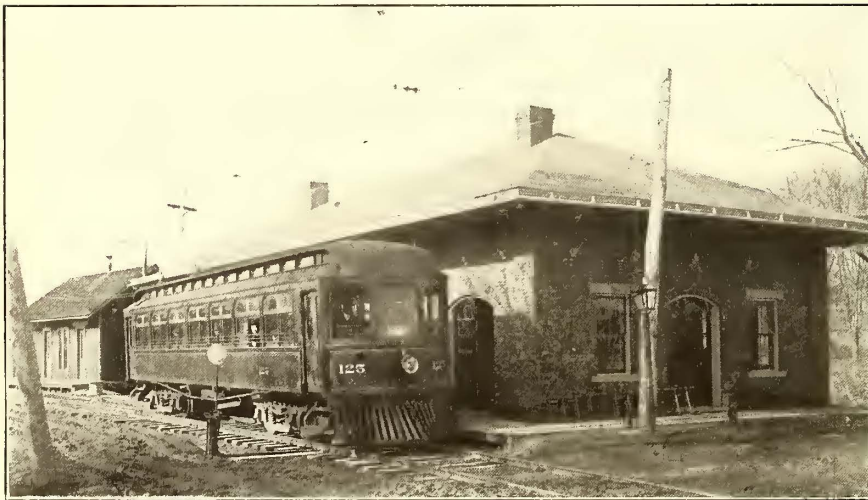
MOUNT WASHINGTON SUB-STATION AND PASSENGER DEPOT
