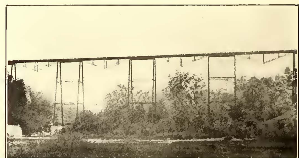
STEEL TRESTLE 110 FT. ABOVE WATER
