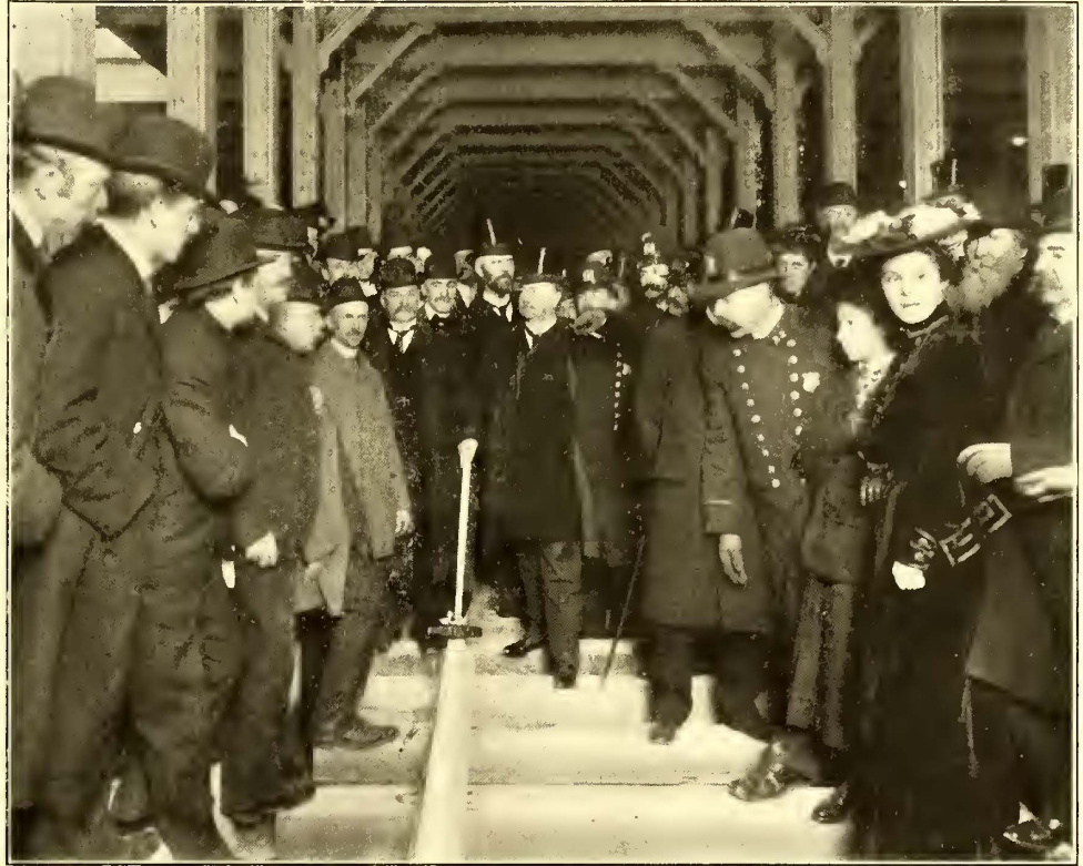
MAYOR LOW DRIVING FIRST SPIKE IN SUBWAY TRACK, MARCH 14
