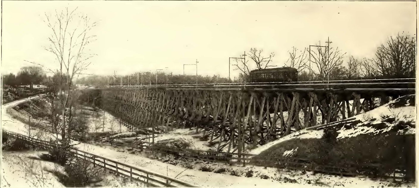
TRESTLE AT SLATE HILL NEAR ENTRANCE TO GLENMARY PARK
