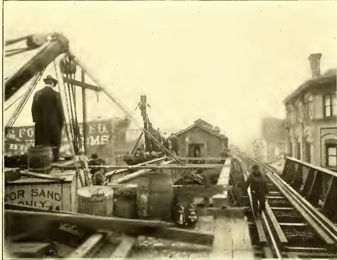
SOUTHBOUND TRACK COMPLETED
