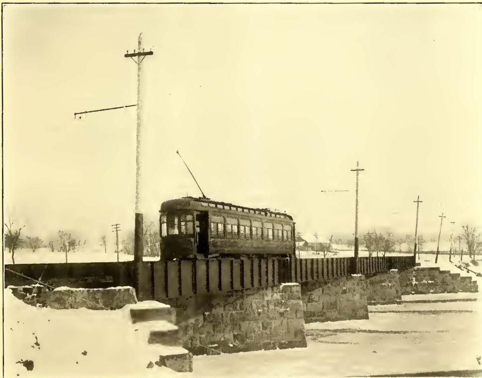
STEEL BRIDGE AT STRATFORD
