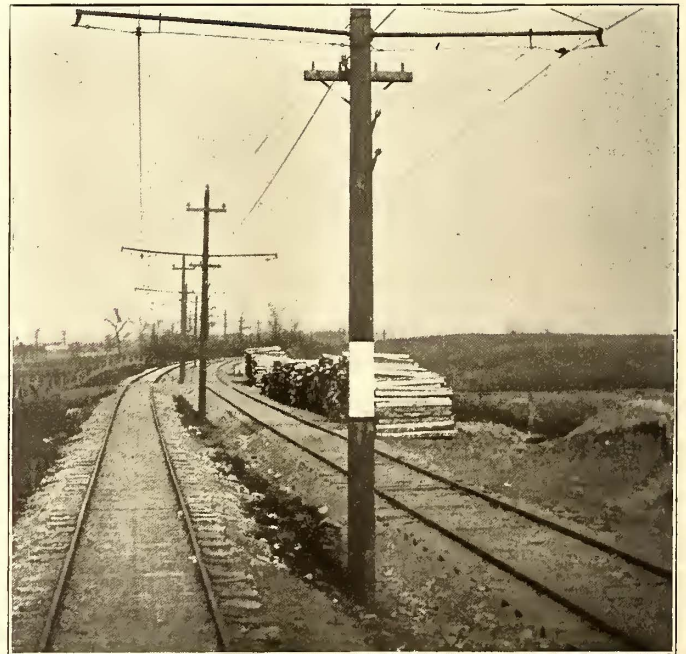
OVERHEAD WORK AT DOUBLE-TRACK CURVE, C., L. & S.
