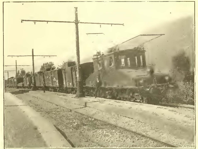
FIG. 19.—DOUBLE-BRACKET CONSTRUCTION
