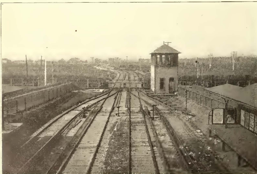
FIG. 3.—VIEW FROM BRIDGE, LOOKING WEST, SHOWING INTERLOCKING TOWER
