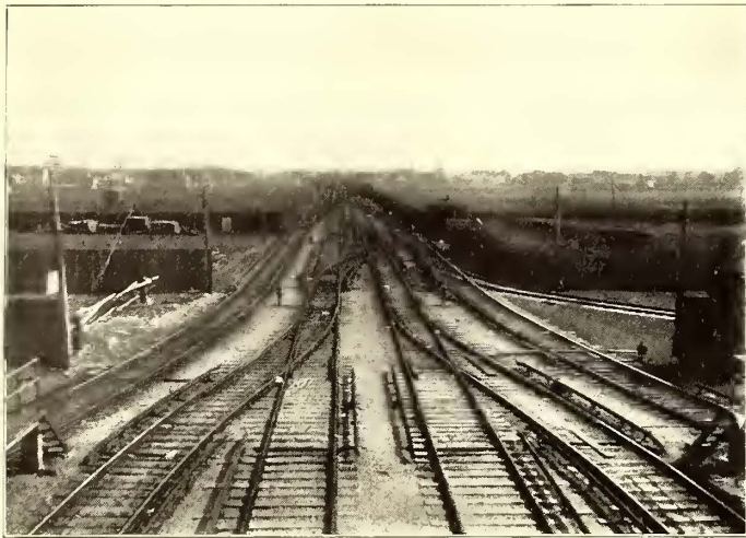
FIG. 7.—LOOKING UP THE INCLINE
