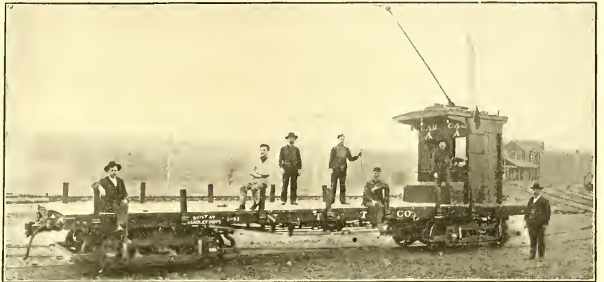
WORK CAR AND CREW
