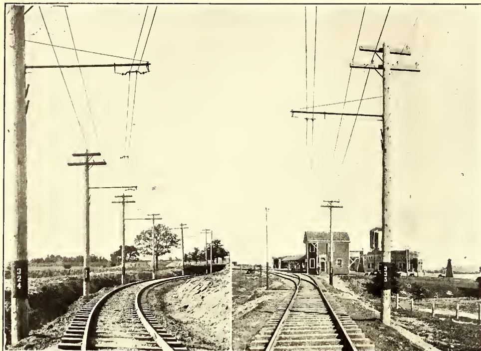
EXAMPLES OF TRACK AND OVERHEAD CONSTRUCTION
